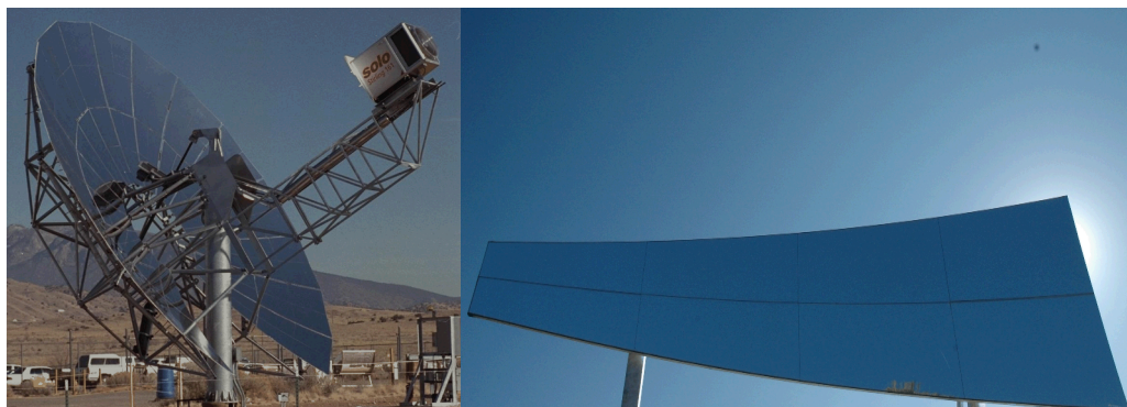
Figure 4. Sandia 10-kWe dish/String system dish system. The structural honeycomb facets have slope errors in the range of 0.8 - 1.4 mrad.
