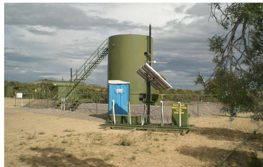
Separator, Produced Water Tank from Well, Shower, Flush Toilet and Sauna ( in blue building)
