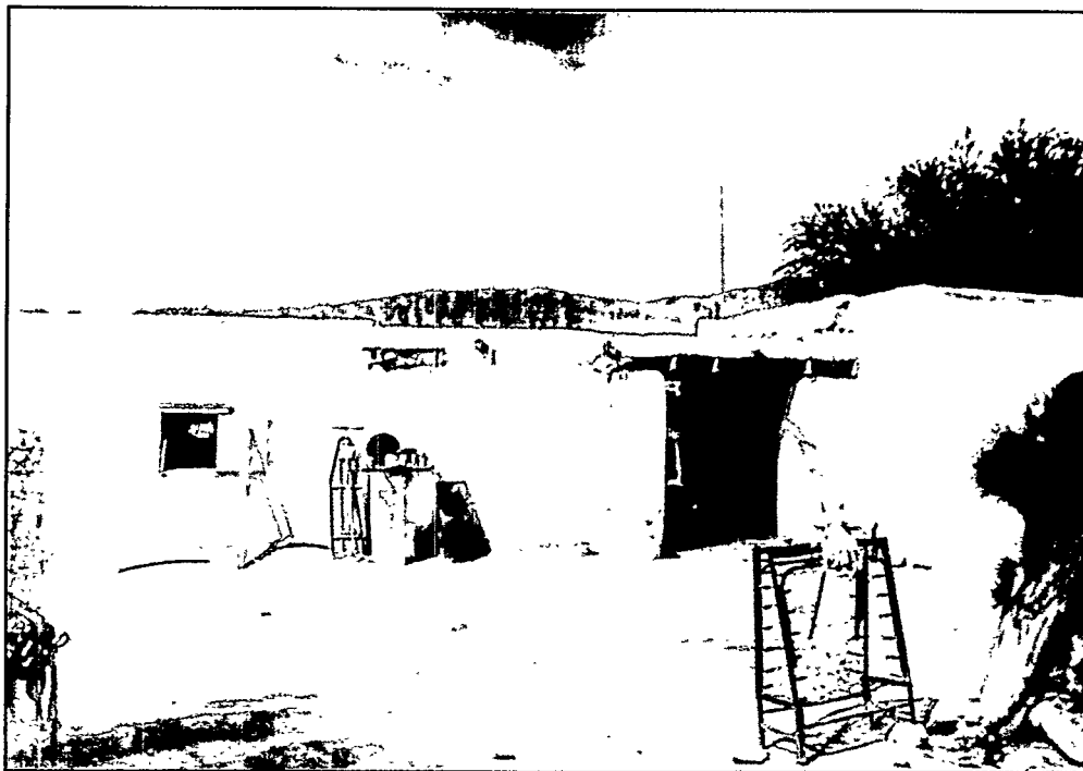
Figure 19. Upper Boquillas residence with electrical tie-in (electrical conduit with wires projecting from roof to left of tree) in anticipation of future power service.
