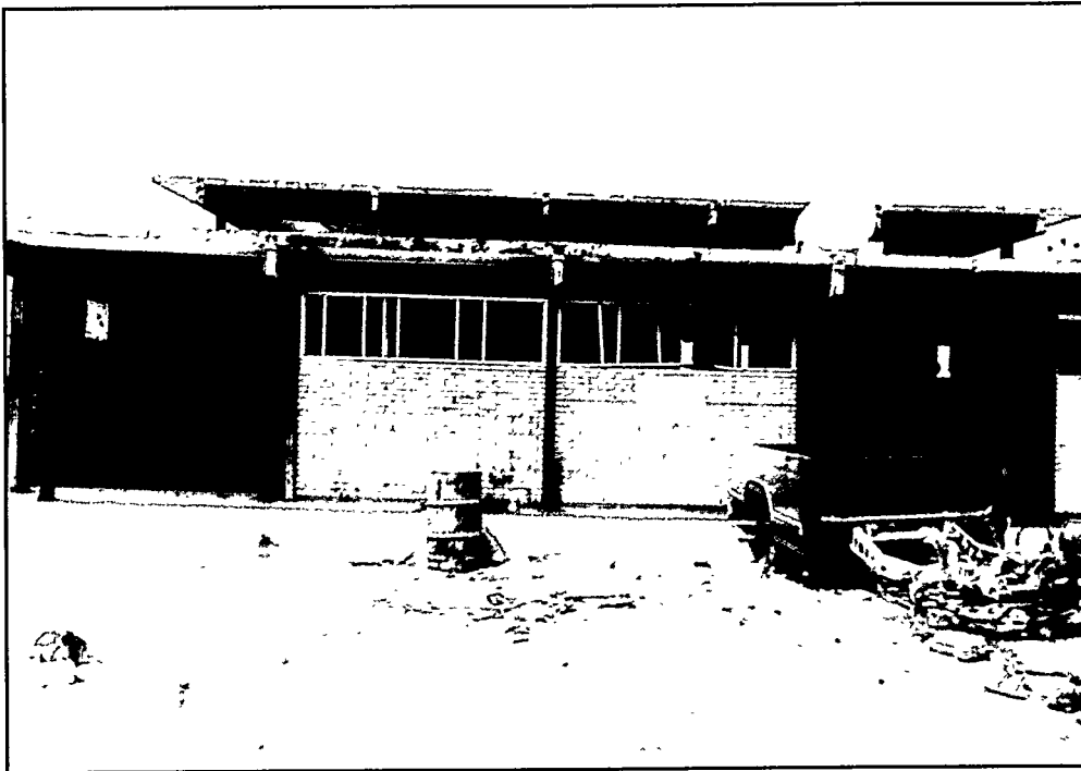
Figure 15. South side of abandoned customs facilities.
