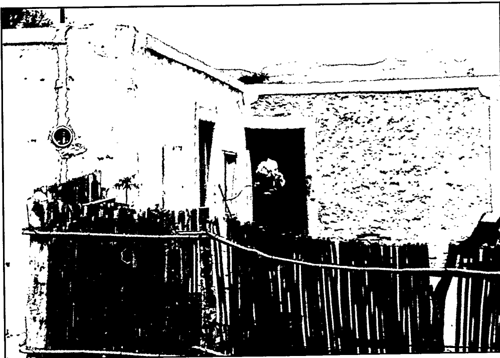
Figure 25. Lower Boquillas residence with propane tank by kitchen; note the electrical conduit projecting from left wall into the skyline with fuse box in wall.
