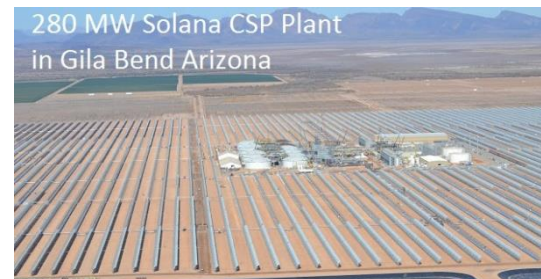
280 MW Solana Parabolic Trough Plant with 6 hours storage, Gila Bend, AZ
