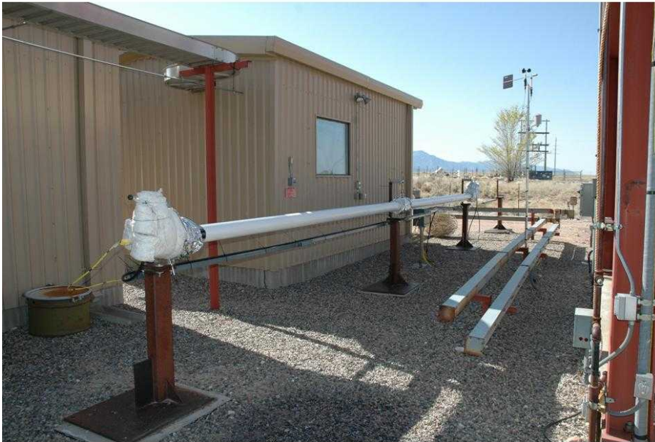
Impedance heating system at SNL
