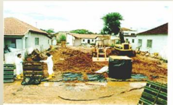
14. The same site after removal of the contaminated rubble.
