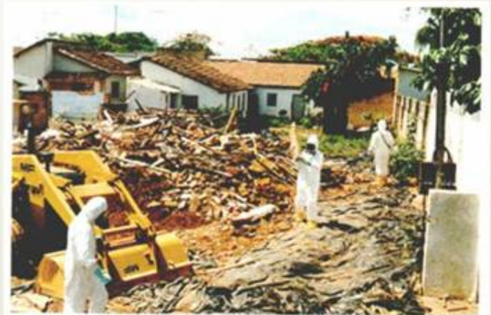
13. Contaminated rubble from the demolition of R.A.'s house on 57th Street.
