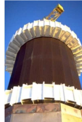
Solar Two Molten Salt Receiver (Pacheco, 2002)
