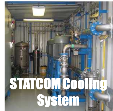
Thyristor Cooling Pipes
