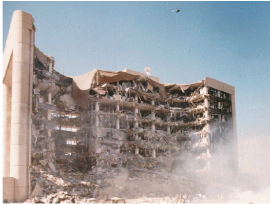
blast induced structural collapse
