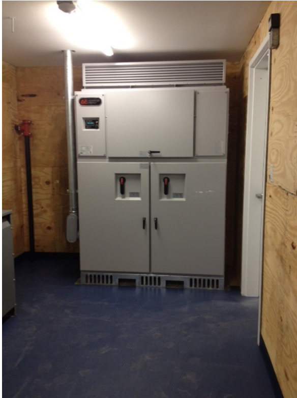
Advanced Energy AE 100TX Three-phase Inverter installed at U.S.S Juneau Memorial Center, Kearny, NJ
