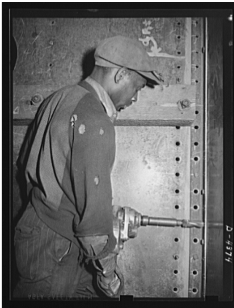
Figure 7: "Manpower. Negro shipyard workers. American manpower draws its skills from all citizens alike. This Negro power drill operator is reaming a hole through which rivets will be driven in the building of warships in an Eastern shipyard. Federal Shipbuilding and Drydock Corporation. Kearny, New Jersey." Source: Library of Congress, Farm Security Administration - Office of War Information Photograph Collection. Federal Shipbuilding and Drydock Corporation; Howard Liberman, photographer, May 1942. Reproduction Number: LC-USE6-D-004374 (b&w film neg.)
