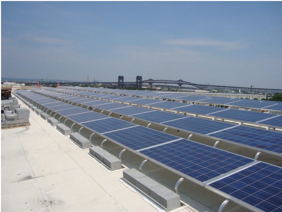
Installation of 364 Sharp ND-U230Q1 photovoltaic panels on roof of Hudson County Juneau Memorial Center
