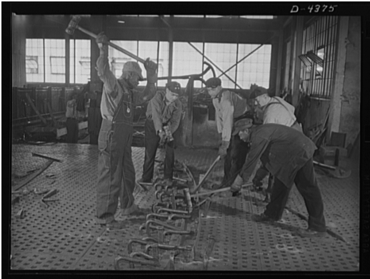
Figure 9: "Manpower. Negro shipyard workers. The hammer is still an important tool in ship production. These workers are bending metal fittings on a furnace slab floor, an operation in ship construction at a large Eastern yard. Federal Shipbuilding and Drydock Corporation. Kearny, New Jersey." Source: Library of Congress, Farm Security Administration - Office of War Information Photograph Collection. Federal Shipbuilding and Drydock Corporation; Howard Liberman, photographer, May 1942. Reproduction Number: LC-USE6-D-004375 (b&w film neg.)
