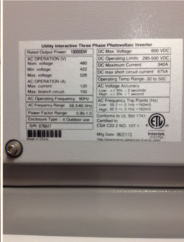
Advanced Energy AE 100TX Three-phase Inverter installed at U.S.S Juneau Memorial Center, Kearny, NJ
