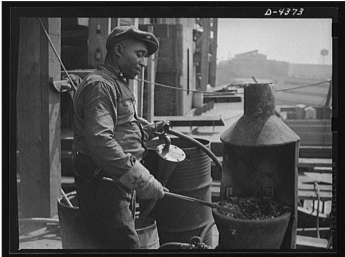
Figure 8: "Manpower. Negro shipyard workers. A hot one for Hitler. This worker heats the rivets which go into Uncle Sam's mighty warships being produced in a large Eastern shipyard. Federal Shipbuilding and Drydock Corporation. Kearny, New Jersey." Source: Library of Congress, Farm Security Administration - Office of War Information Photograph Collection. Federal Shipbuilding and Drydock Corporation; Howard Liberman, photographer, May 1942. Reproduction Number: LC-USE6-D-004374 (b&w film neg.)
