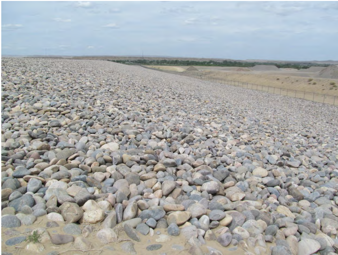
SHP 5/2013. PL-10. Southeast slope of disposal cell.
