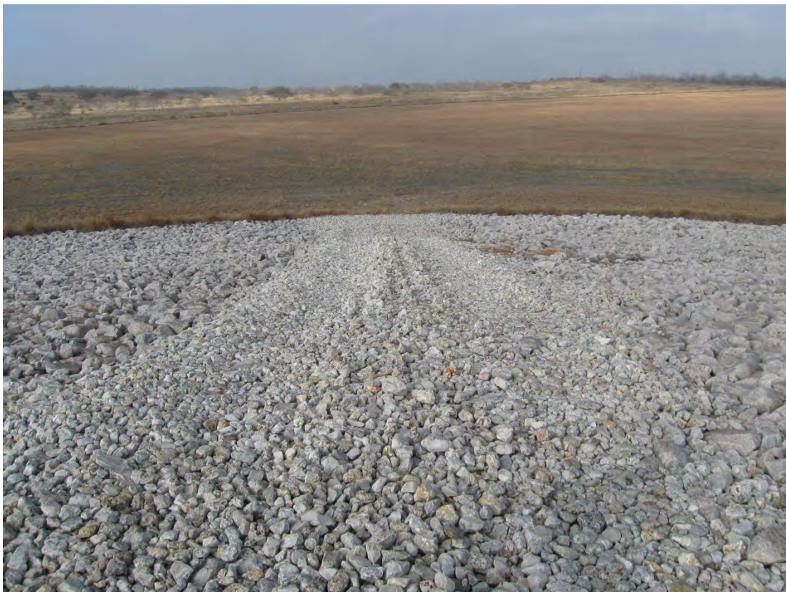
FCT 1/2013. PL-9. Ramp on west corner of cell.
