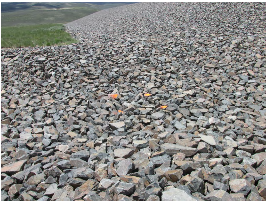
GUD 6/2013. PL-10. Riprap test area No. 4 in the east diversion channel.
