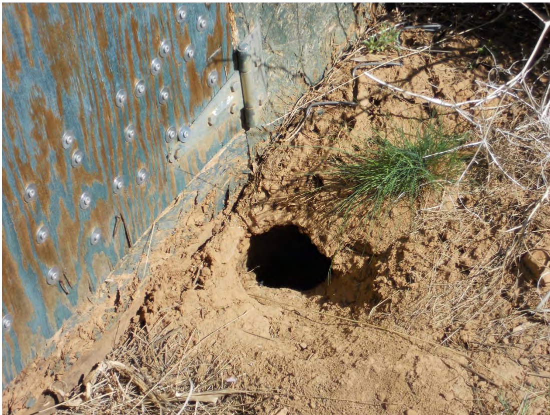
DUD 5/2013. PL-14. Animal burrow under east side (front) of shed. Edge of pond liner is at top of photo.
