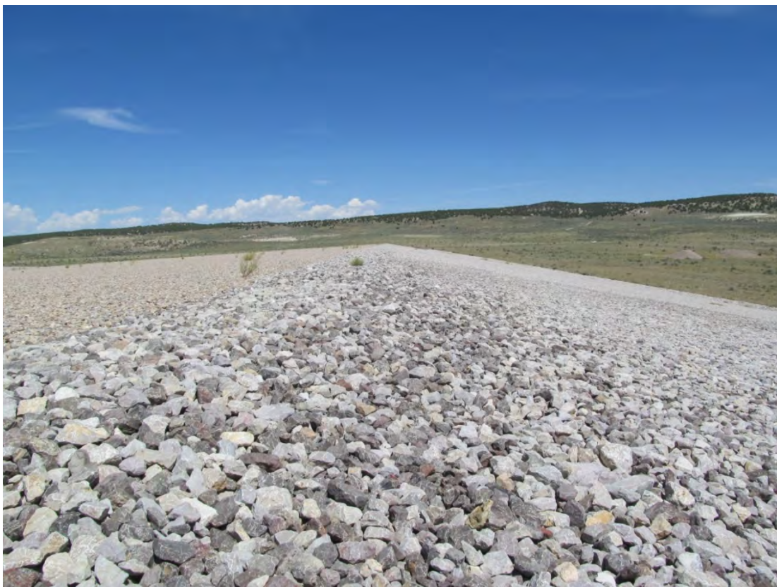
MAY 8/2013. PL-6. Northeastern edge of the disposal cell top.
