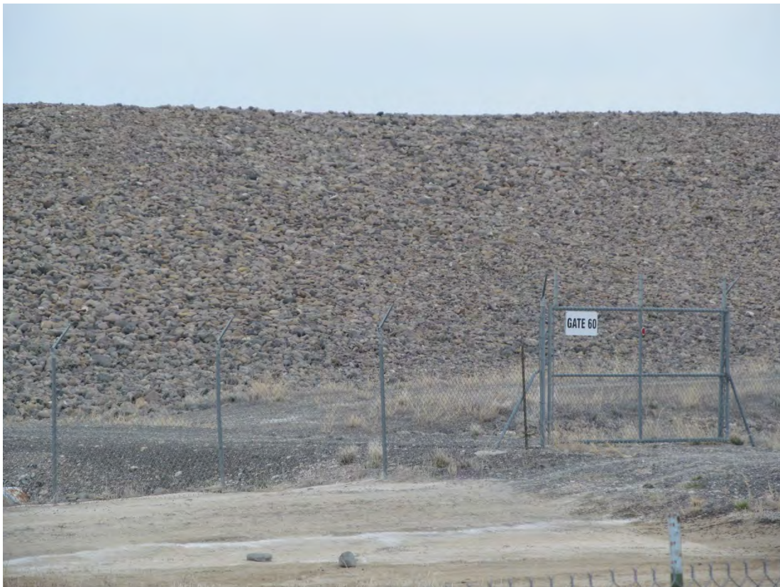
SLD 3/2013. PL-1. Southwest corner from outside fence surrounding the cell.
