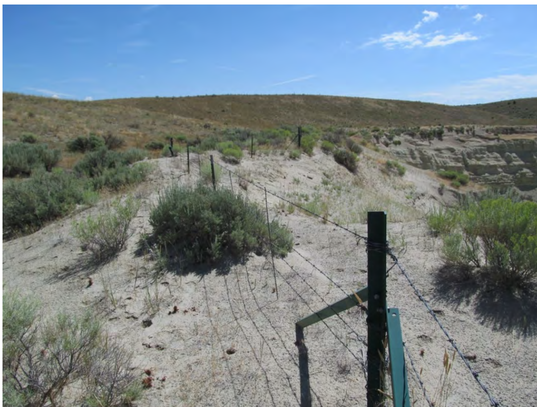
MAY 8/2013. PL-12. Windblown sand accumulation along the south perimeter fence at crest of the northern wall of the Johnson Pit; encroachment of pit in background.
