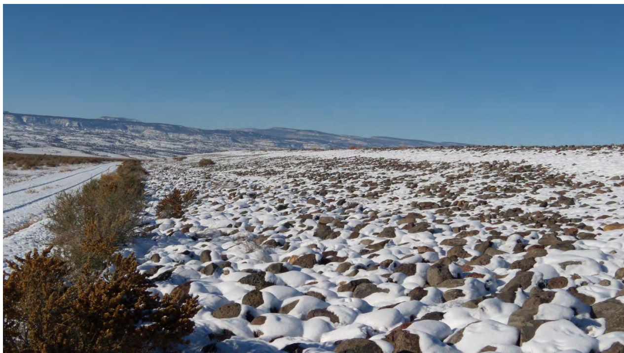
GRJ 12/2013. PL-6. South slope of disposal cell.
