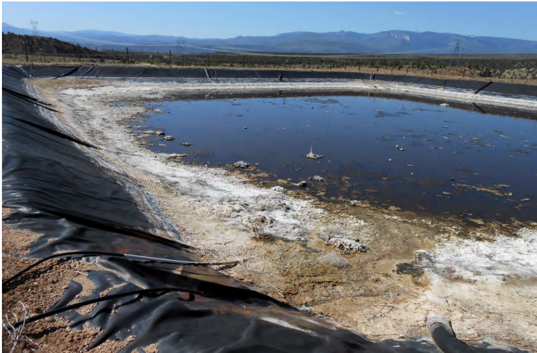
RFL 6/2013. PL-6. Evaporation pond with low water level.
