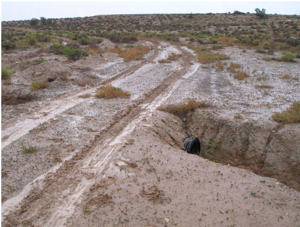
SRK 11/2013 PL-7 Culvert before replacement
