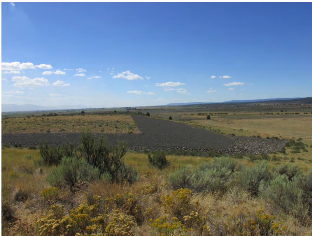
LKV 8/2013. PL-4. View to south across site from north site fence. North and west rock side slopes, and energy dissipation area are shown.
