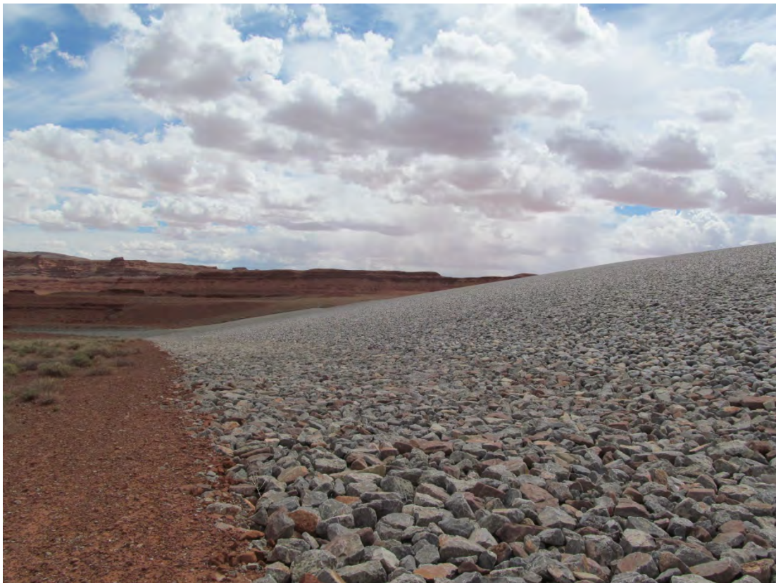
HAT 4/2013. PL-6. North toe drain/northeast side slope.
