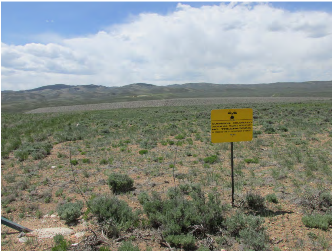
GUD 6/2013. PL-3. Perimeter sign P22 and the disposal cell.
