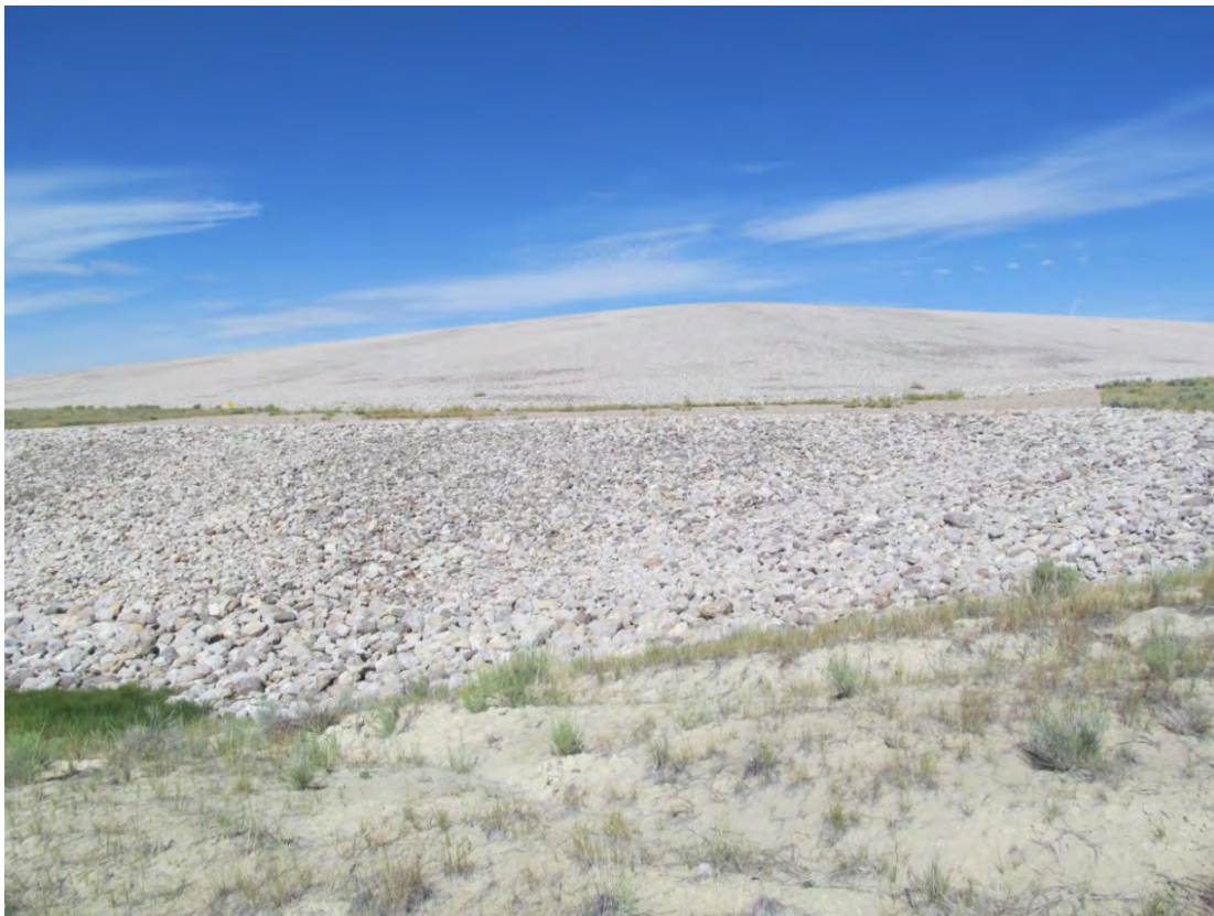
MAY 8/2013. PL-9. Armored Gully No. 1; disposal cell in background.
