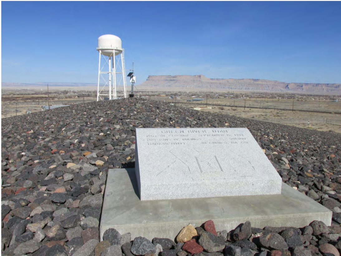
GRN 3/2013. PL-4. Site marker SMK-2 on the disposal cell crest.
