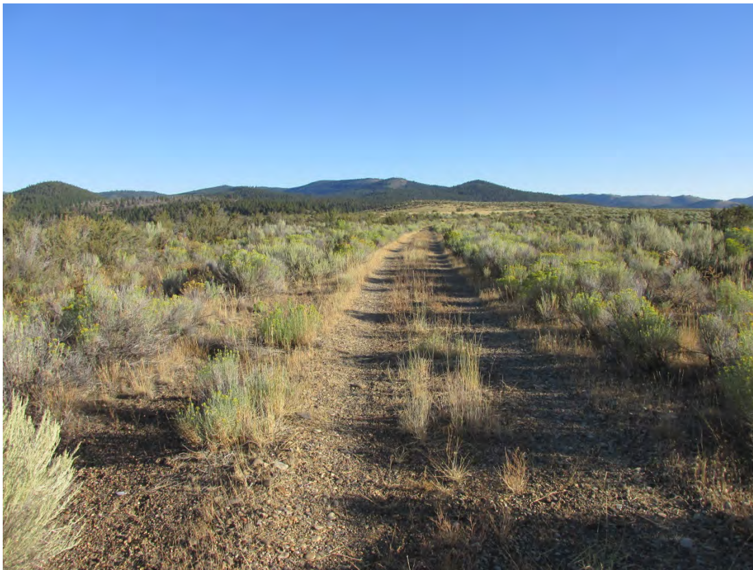
LKV 8/2013. PL-1. Gravel site access road. View to north.
