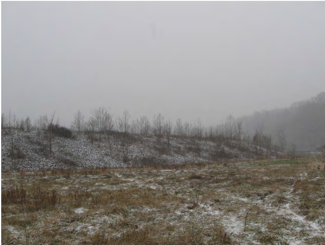
BUR 12/2013. PL-10. Northeast face of disposal cell.
