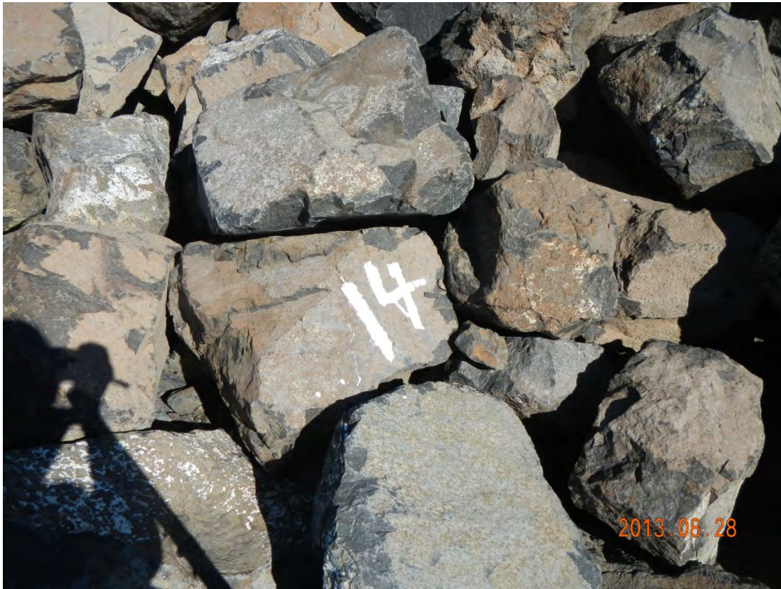
LKV 8/2013. PL-8. Riprap photo-monitoring location 14 in EDA.
