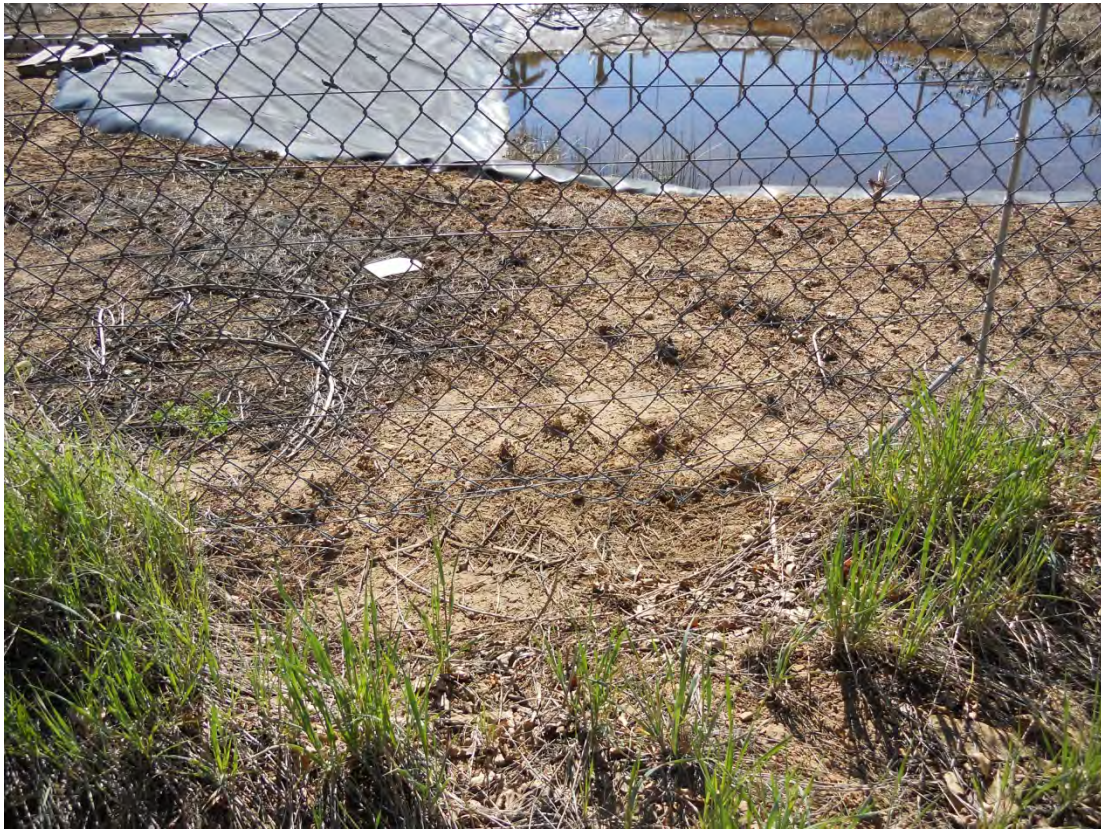
DUD 5/2013. PL-15. Gap under evaporation pond fence, west side.
