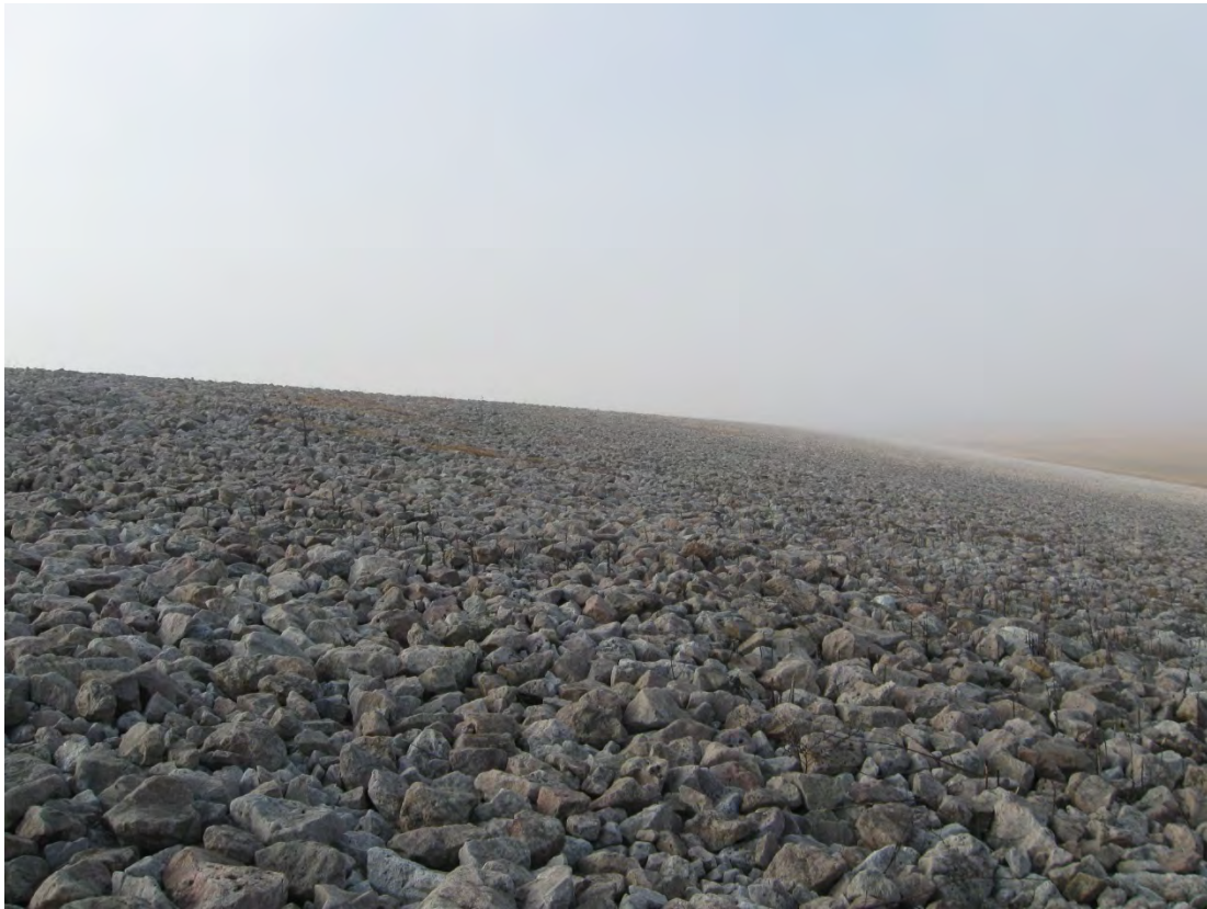
FCT 1/2013. PL-6. Looking southwest down northwest side slope.
