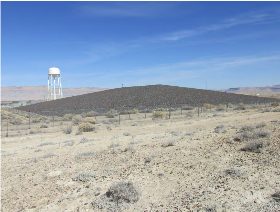
GRN 3/2013. PL-5. Disposal cell.
