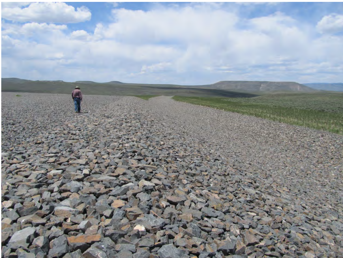
GUD 6/2013. PL-8. Northwest side of the disposal cell and the west diversion channel.
