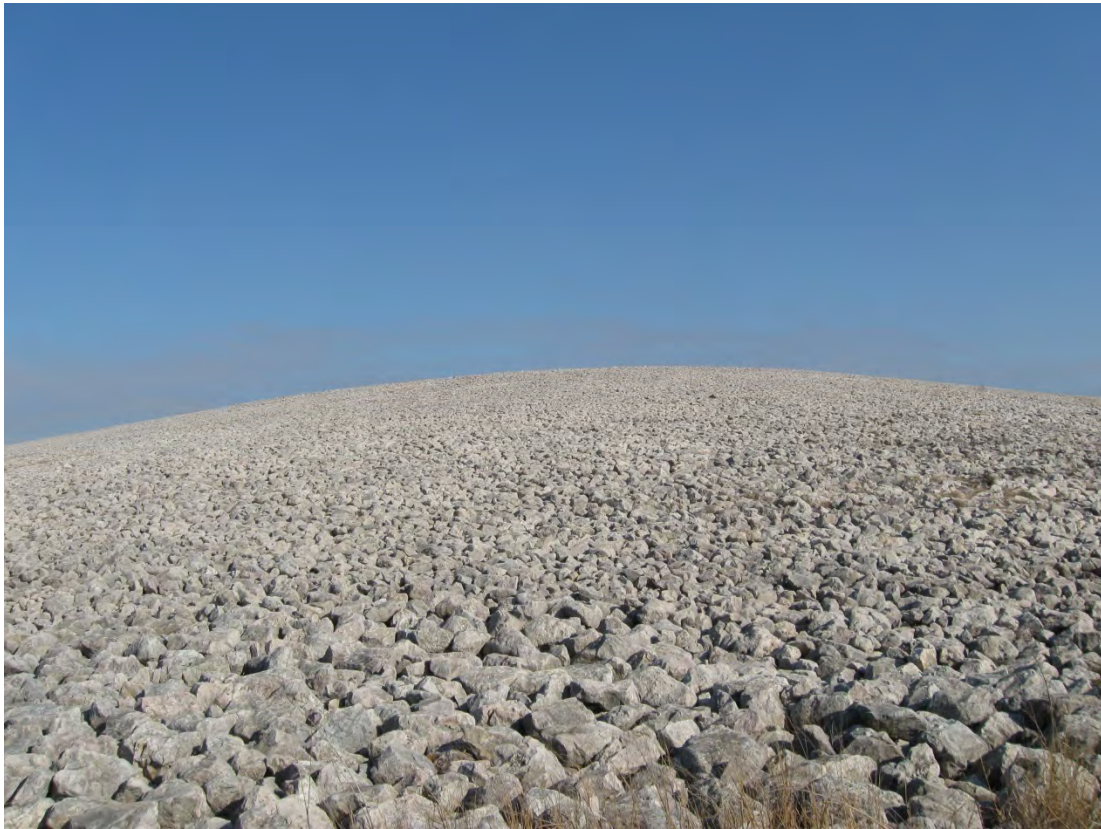
FCT 1/2013. PL-10. Looking up south corner of cell.
