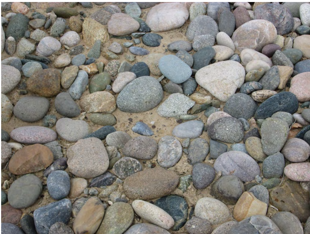
SHP 5/2013. PL-12. Sediment deposition on cell top.
