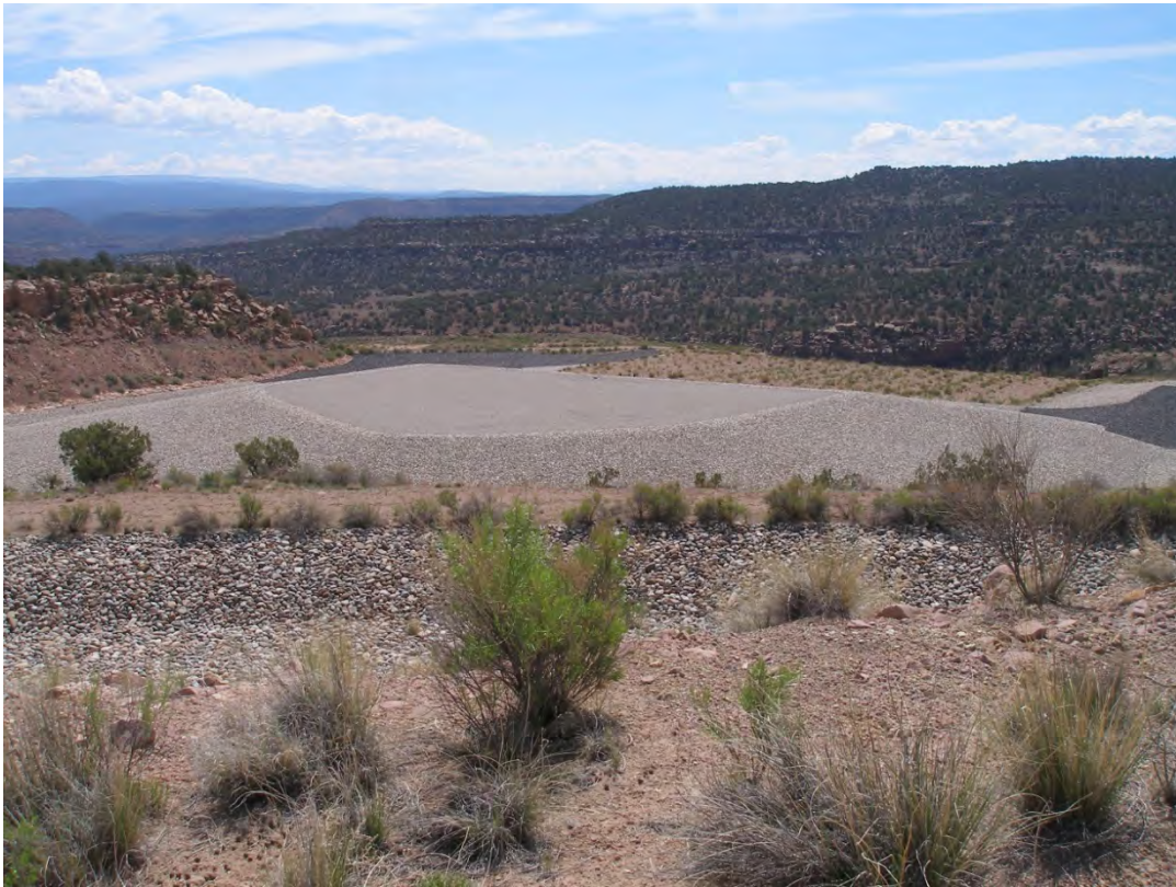
NAD 5/2013. PL-6. View of disposal cell from west-northwest.
