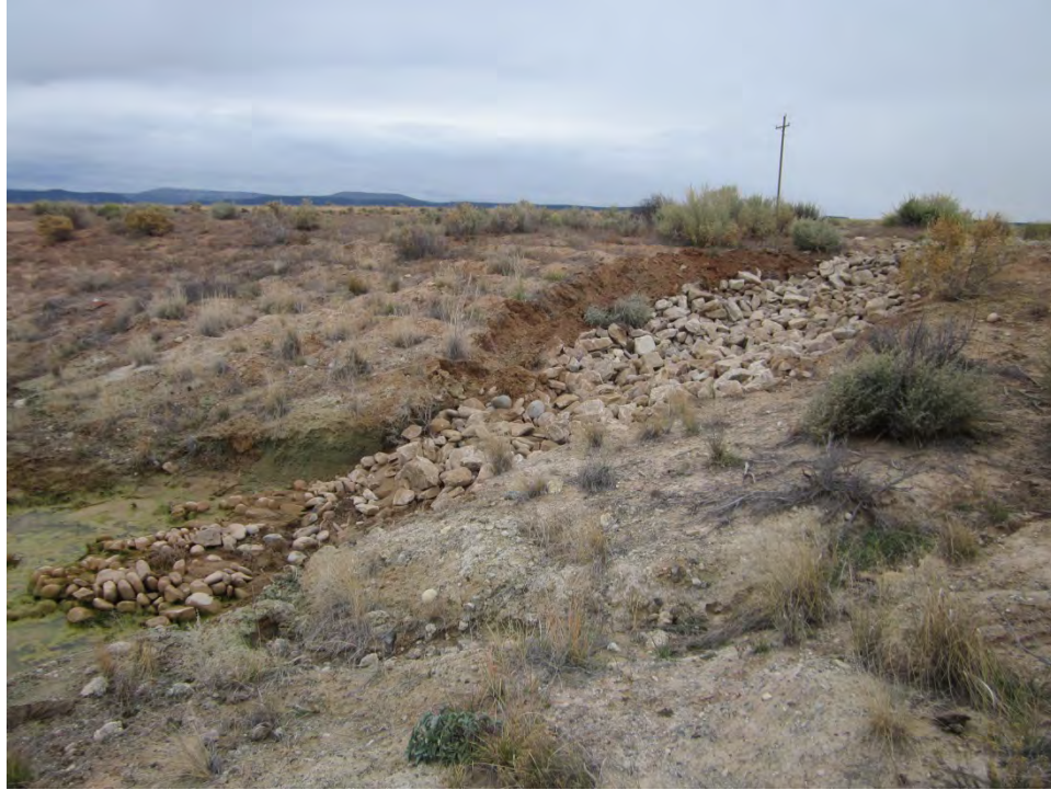
SRK 11/2013 PL-6 Retention pond channel after November repair work.
