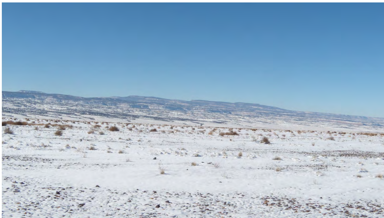
GRJ 12/2013. PL-8. Southwest portion of disposal cell cover.
