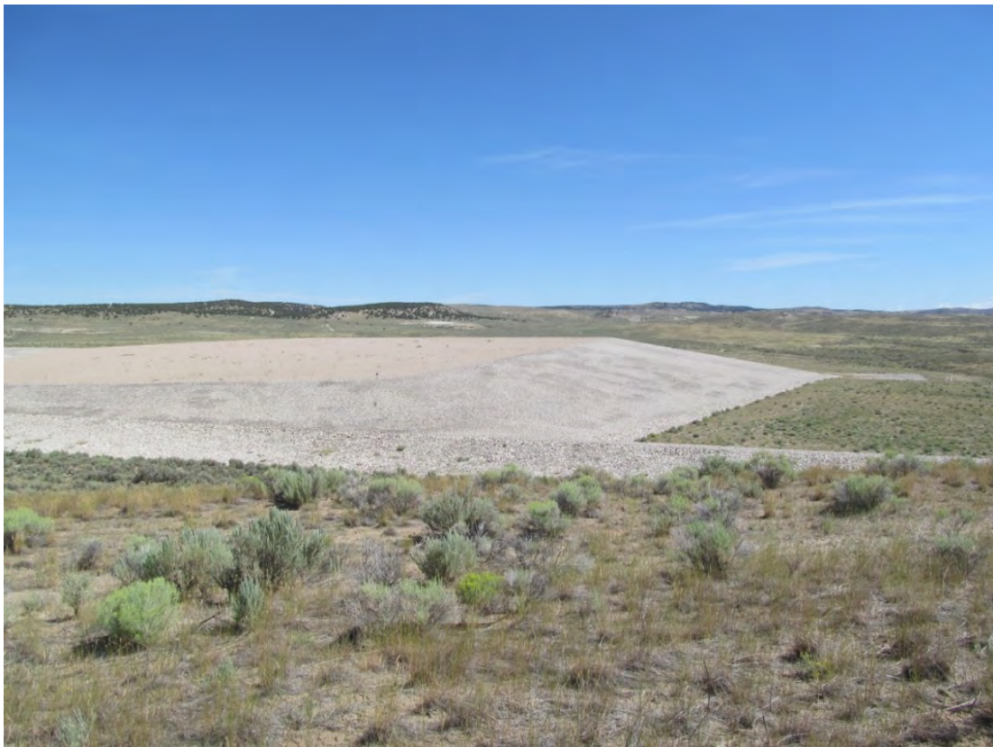
MAY 8/2013. PL-5. Southeastern portion of the disposal cell; Diversion Channel No. 1 in foreground.
