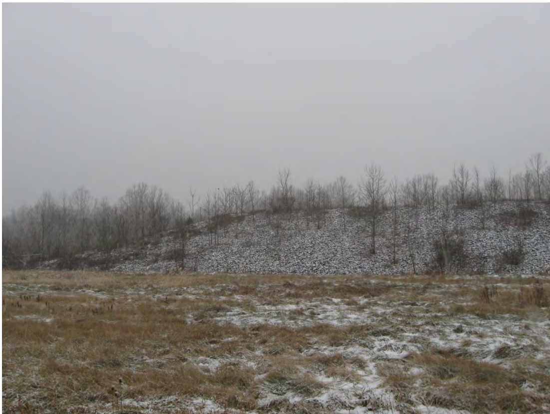
BUR 12/2013. PL-9. Northeast face of disposal cell.
