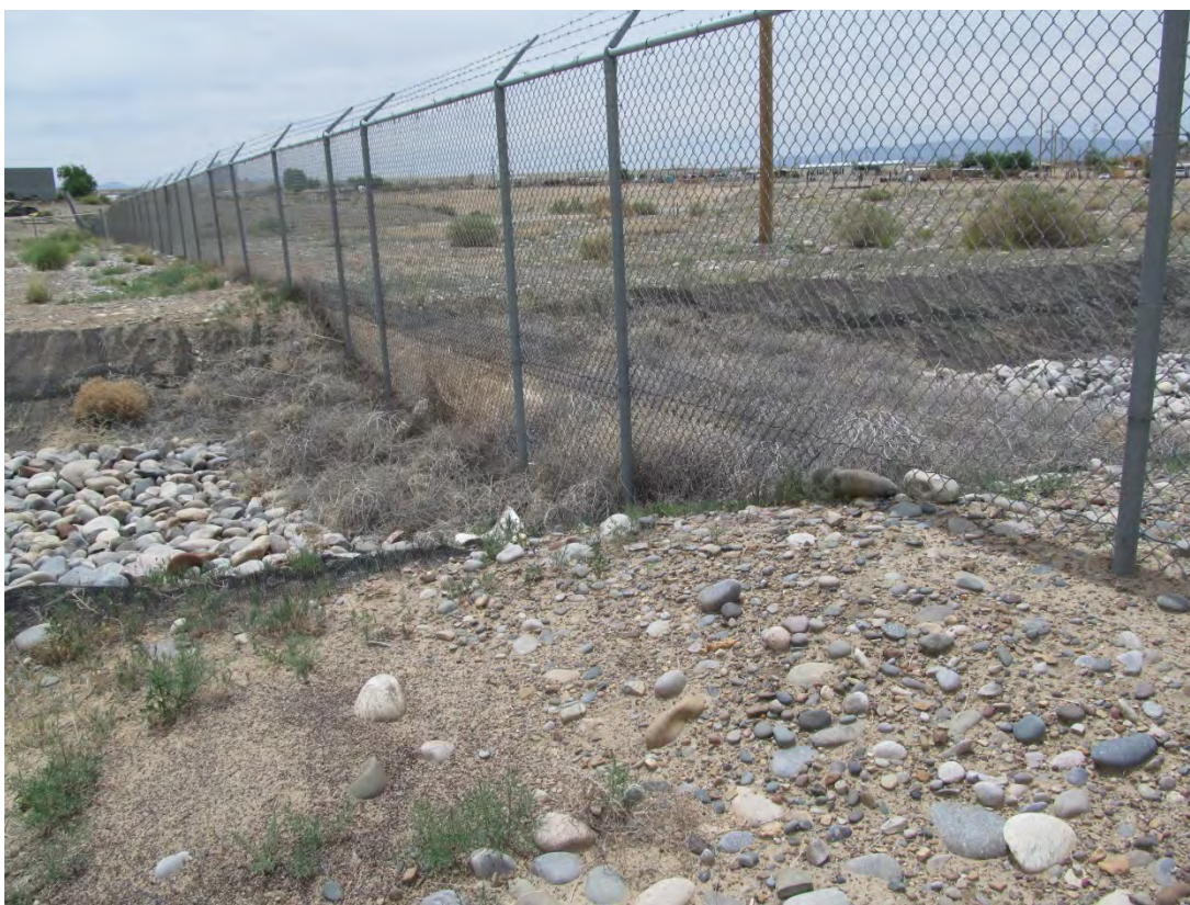
SHP 5/2013. PL-13. Fence across outflow channel with debris buildup.
