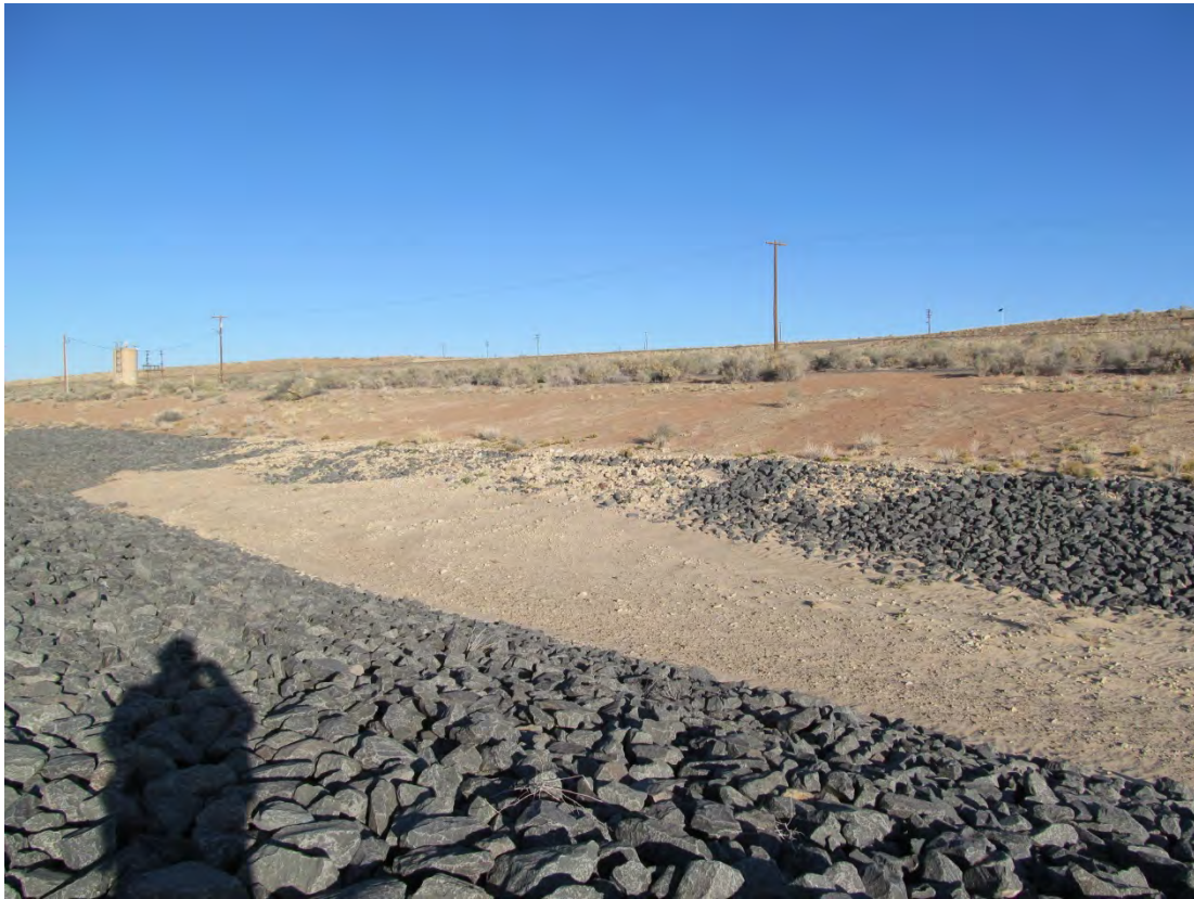
TUB 4/2013. PL-12. Washout and revegetation area.
