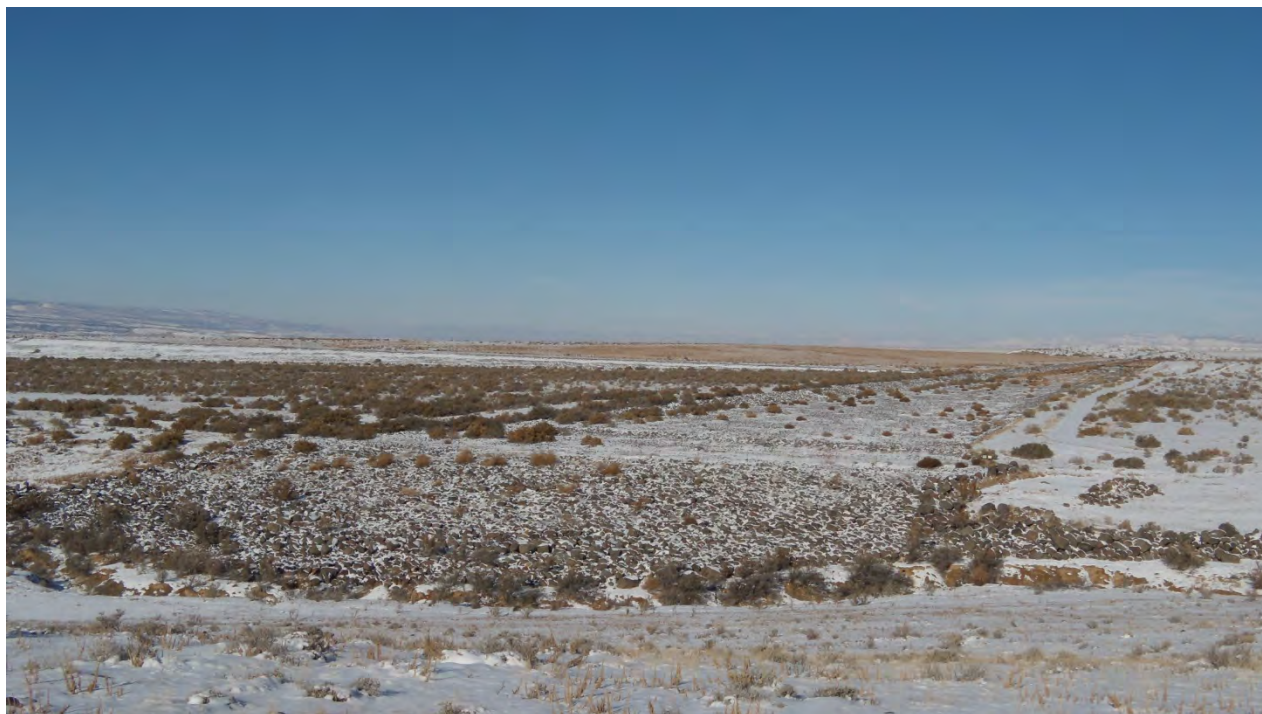
GRJ 12/2013. PL-9. South diversion channel and outlet.
