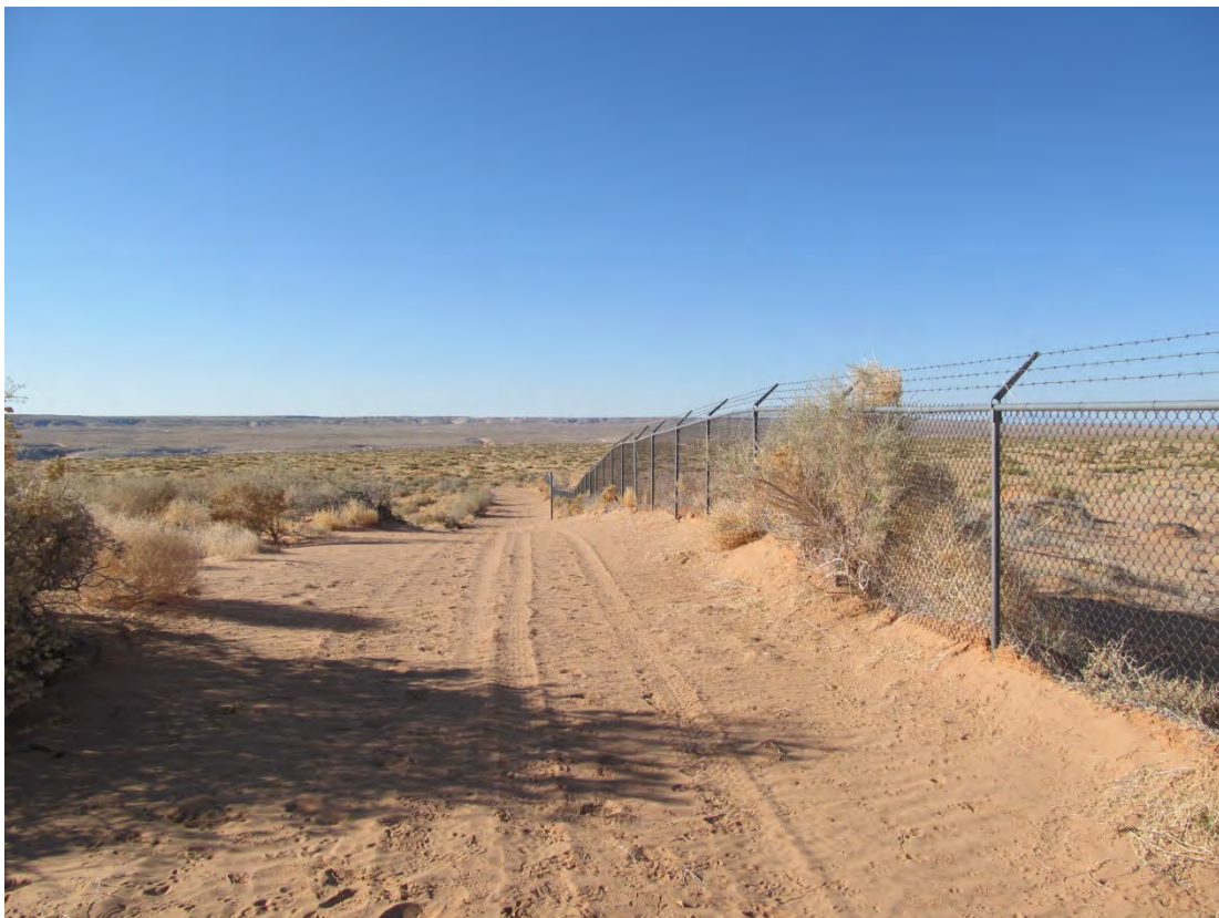
TUB 4/2013. PL-9. Sand accumulation along west boundary fence.
