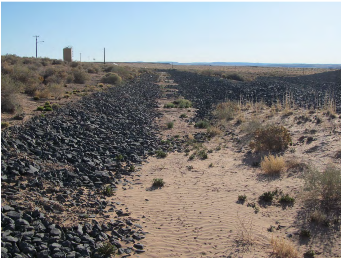
TUB 4/2013. PL-10. East of footbridge showing sediment in channel.
