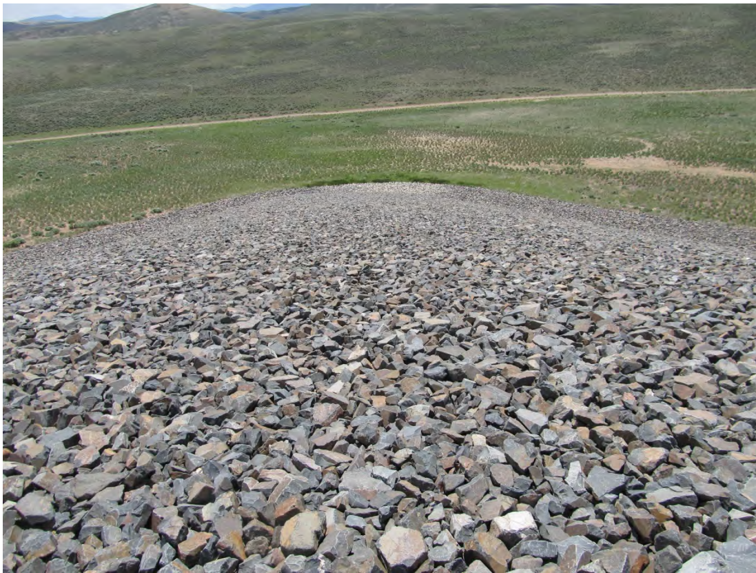
GUD 6/2013. PL-11. Southeast corner of the disposal cell (no runoff water accumulation).
