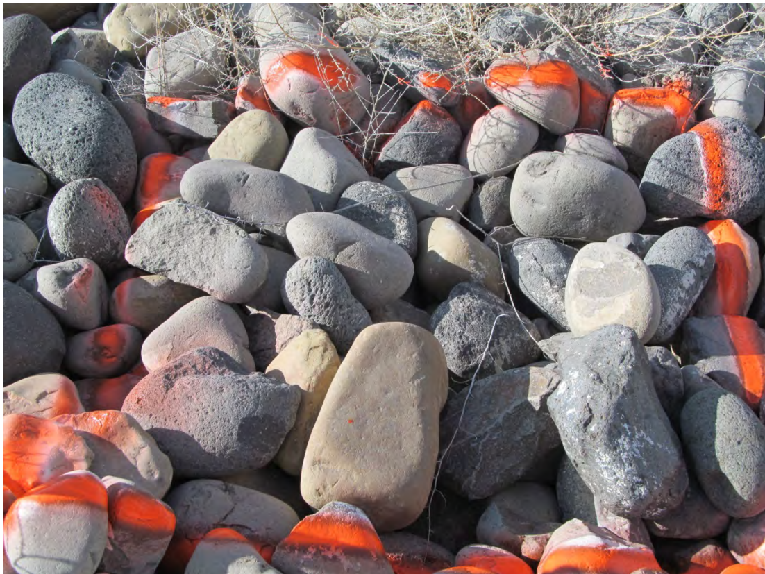
SLD 3/2013. PL-15. Rock Degradation Plot No. 8.
