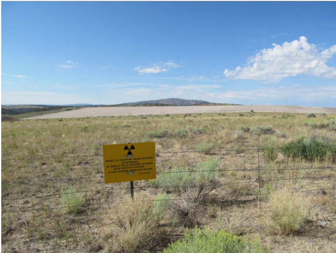
MAY 8/2013. PL-1. Site entrance sign; disposal cell in background.
