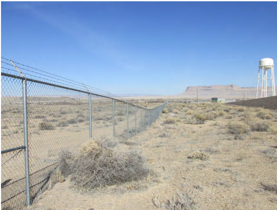
GRN 3/2013. PL-2. Security fence along the southwest side of the disposal cell.
