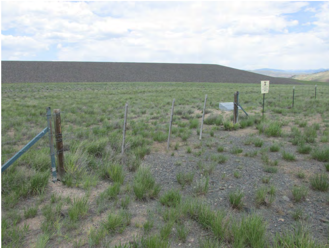
GUD 6/2013. PL-1. Site entrance gate.
