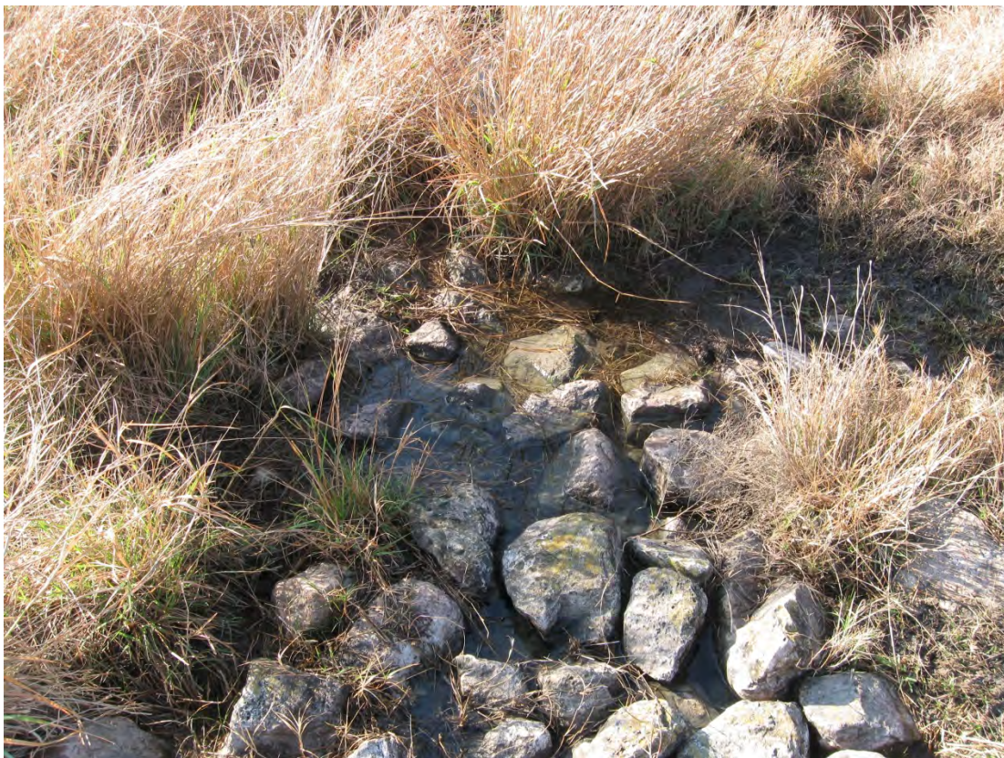
FCT 1/2013. PL-11. Water ponded at outlet of south rock drain.
