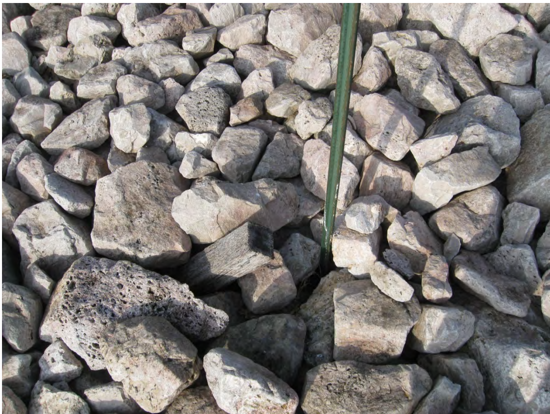
FCT 1/2013. PL-7. Riprap at base of Post 4.
