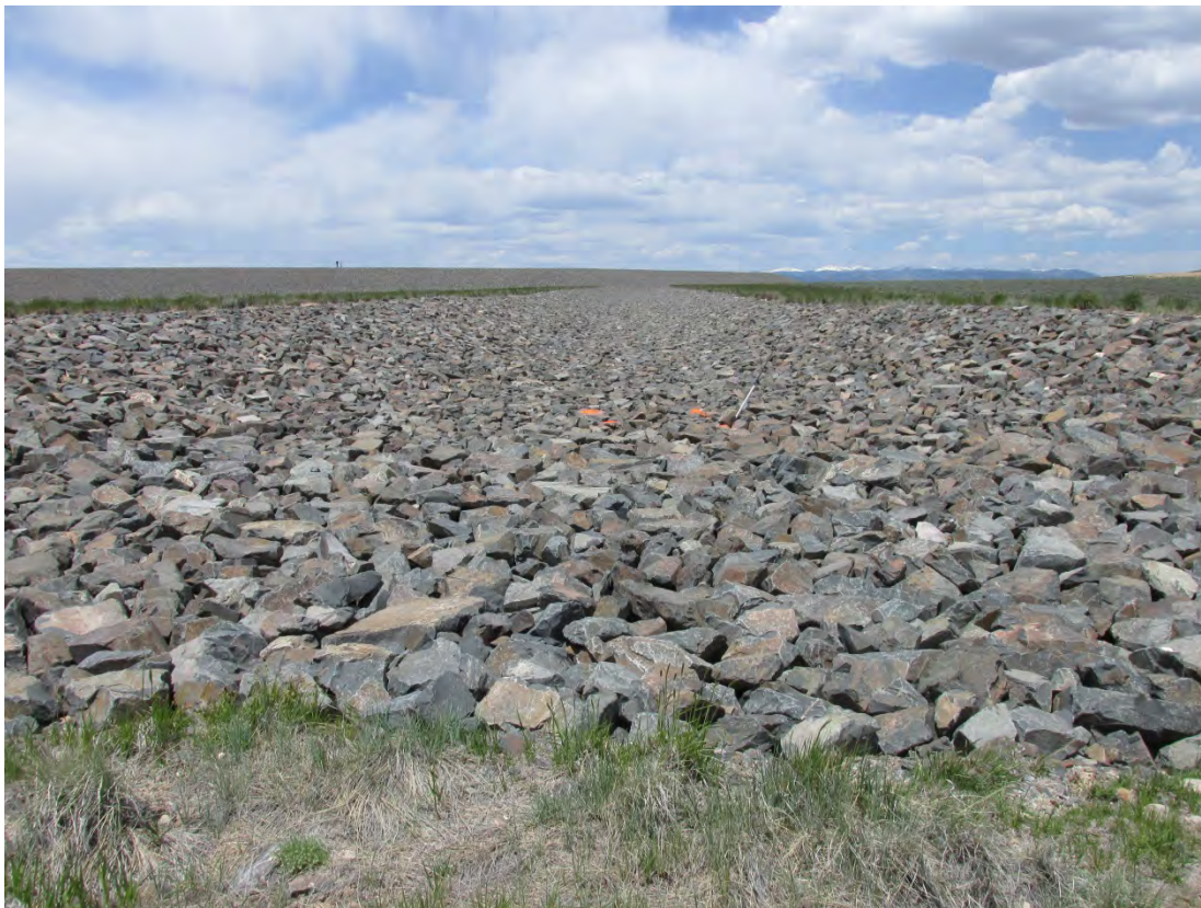
GUD 6/2013. PL-9. View upgradient of the east diversion channel.
