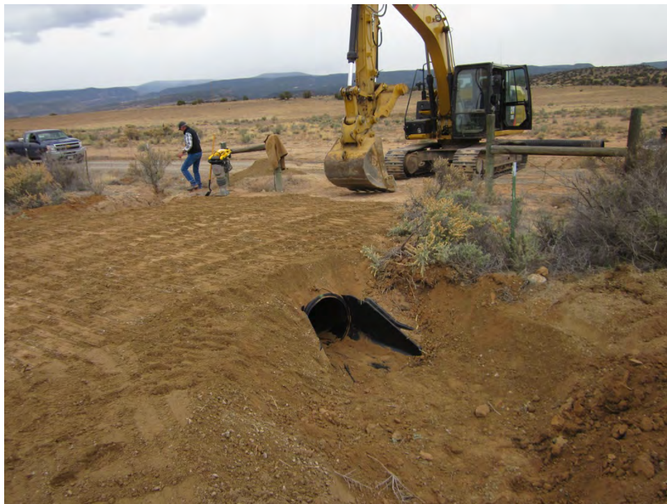
RK 11/2013 PL-8 Culvert after November repairs
