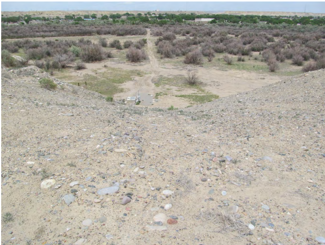
SHP 5/2013. PL-16. View down repaired section of escarpment; no new erosion.
