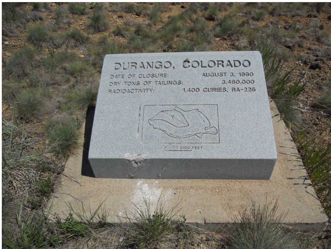
DUD 5/2013. PL-4. Site marker SMK-1, showing damage.
