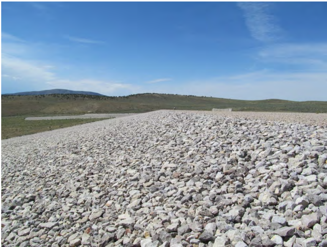
MAY 8/2013. PL-7. Southeastern edge of the disposal cell top.
