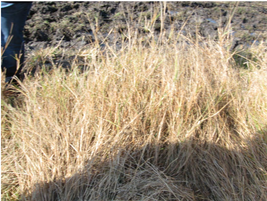
FCT 1/2013. PL-12. Tall grass at outlet of south rock drain.
