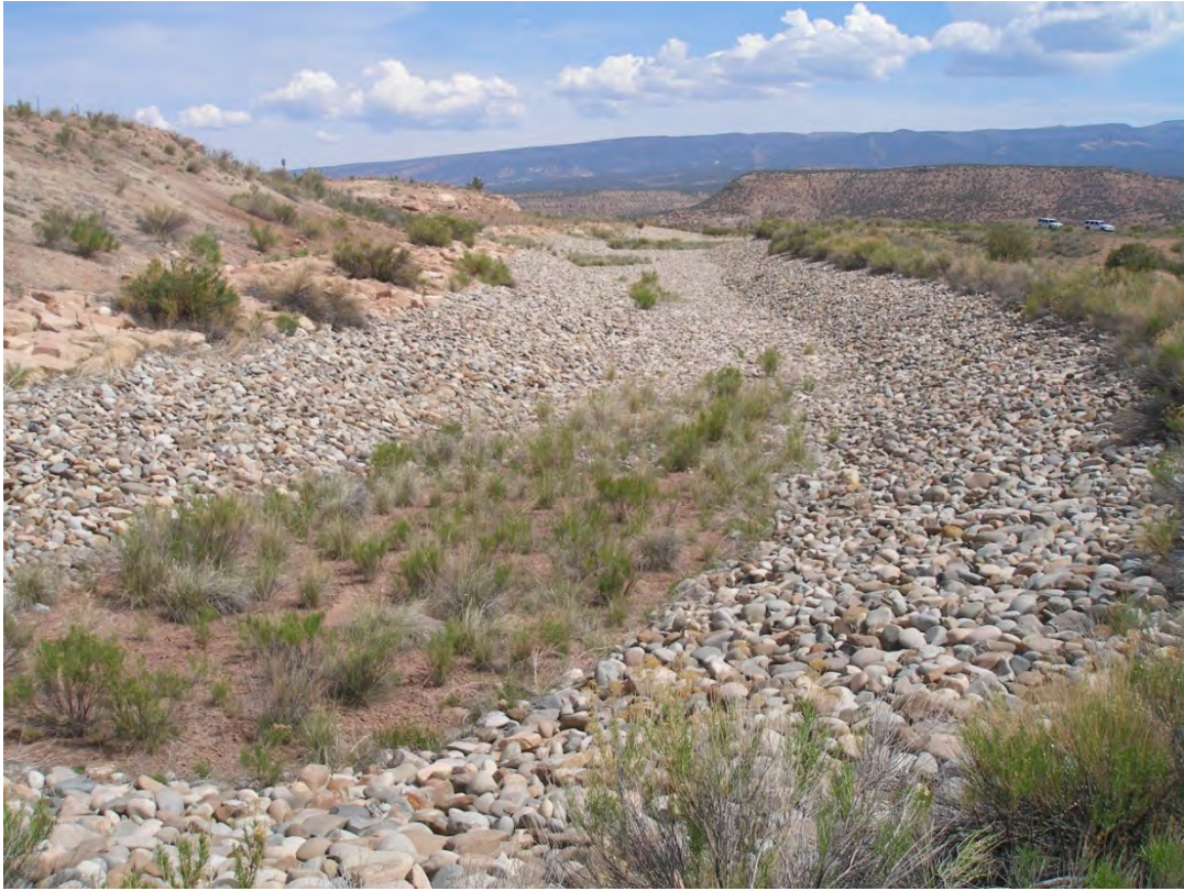
NAD 5/2013. PL-8. View of interceptor channel looking east-northeast.
