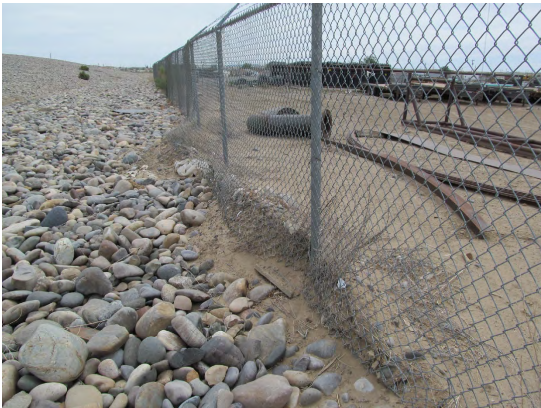
SHP 5/2013. PL-3. Dirt pushed under fence between P11 and P12.
