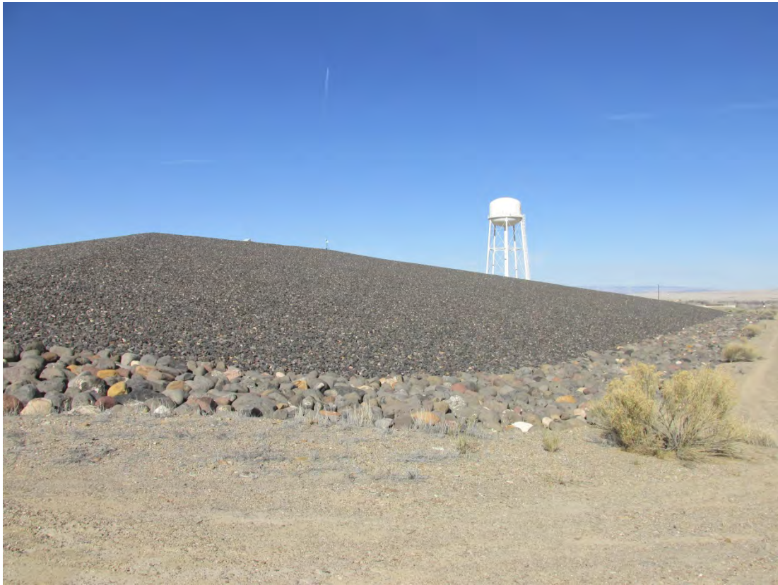
GRN 3/2013. PL-6. Rock apron around the east corner of the disposal cell.
