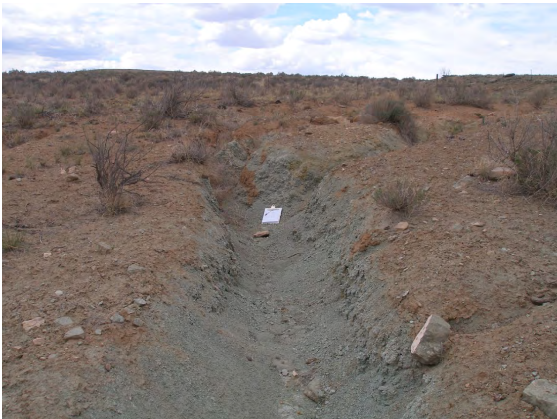
SRK 5/2013. PL-5. Erosion at northwest corner of retention pond.
