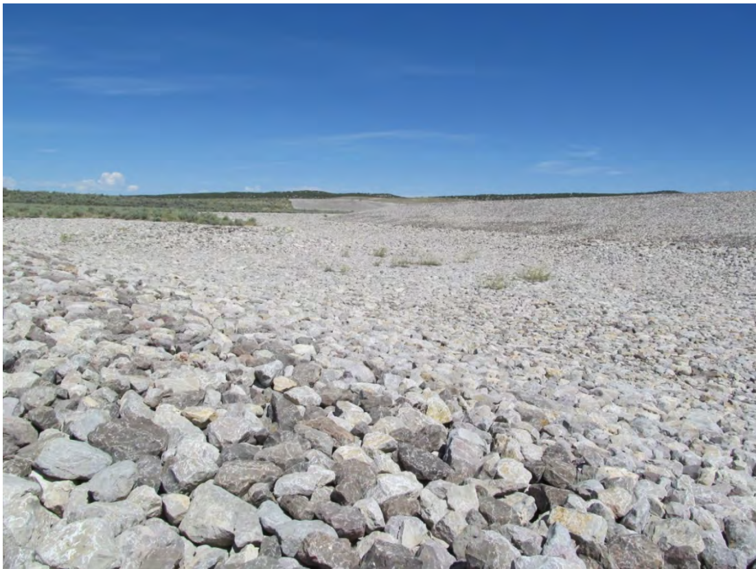
MAY 8/2013. PL-10. Confluence of Diversion Channels No. 1 and 2.
