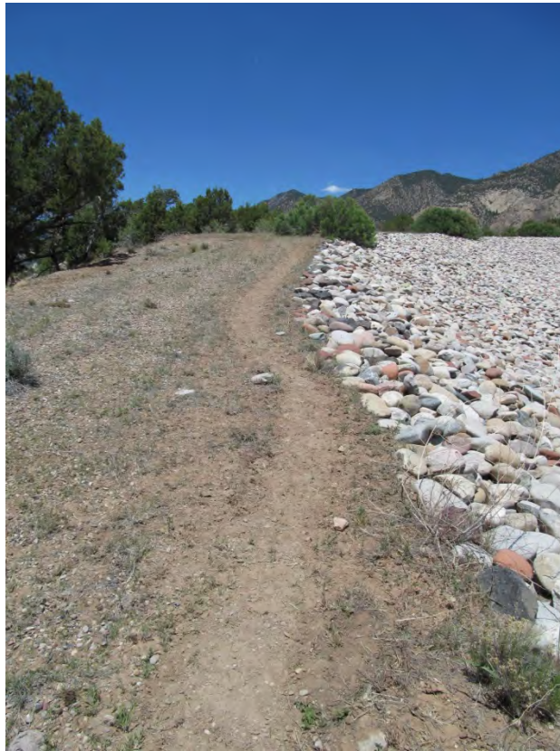
RFL 6/2013. PL-4. Livestock trail along rock riprap cell cover.
