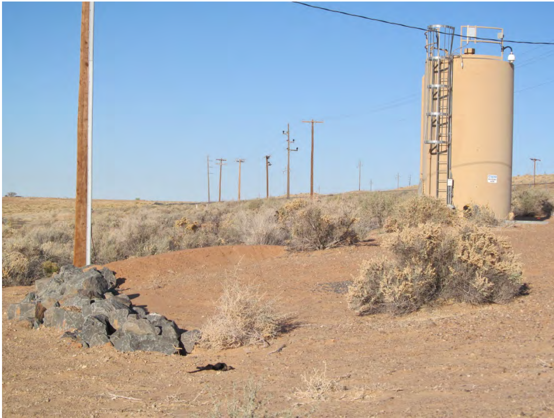
TUB 4/2013. PL-14. Erosion control at distillate tank
