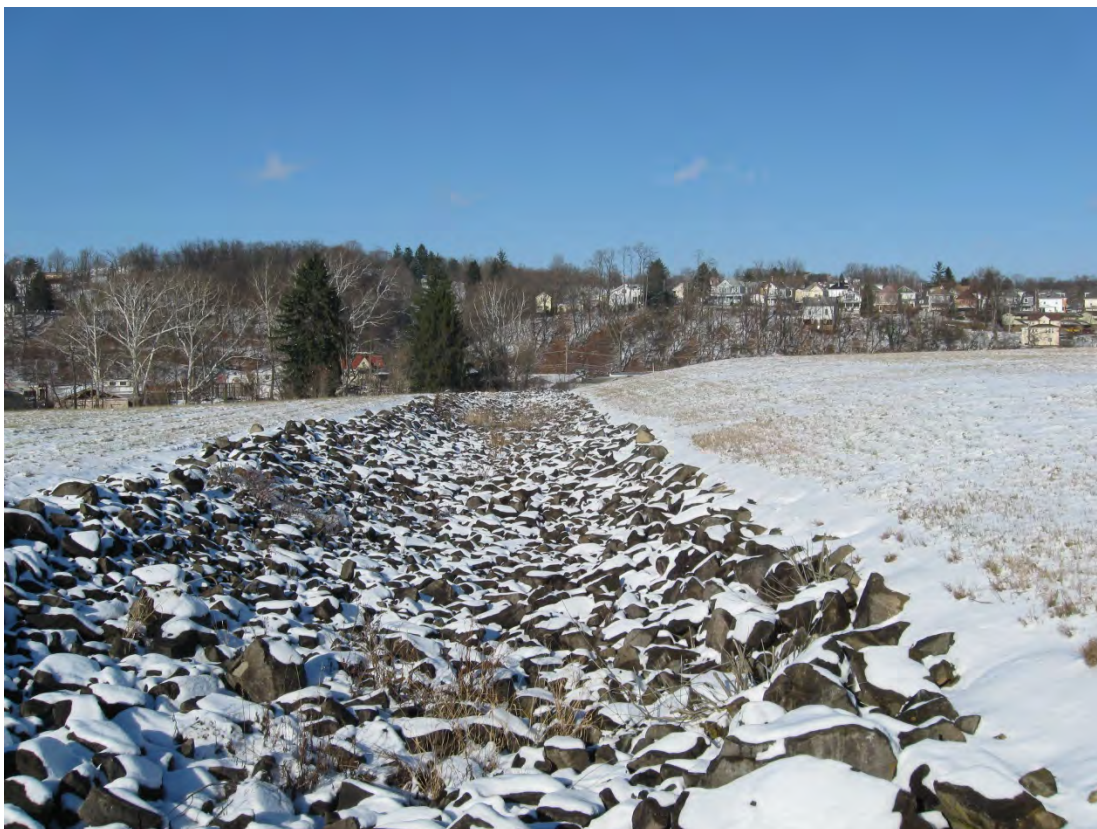
CAN 10/2013. PL-10. Riprap-armored diversion ditch on southwest side of disposal cell.
