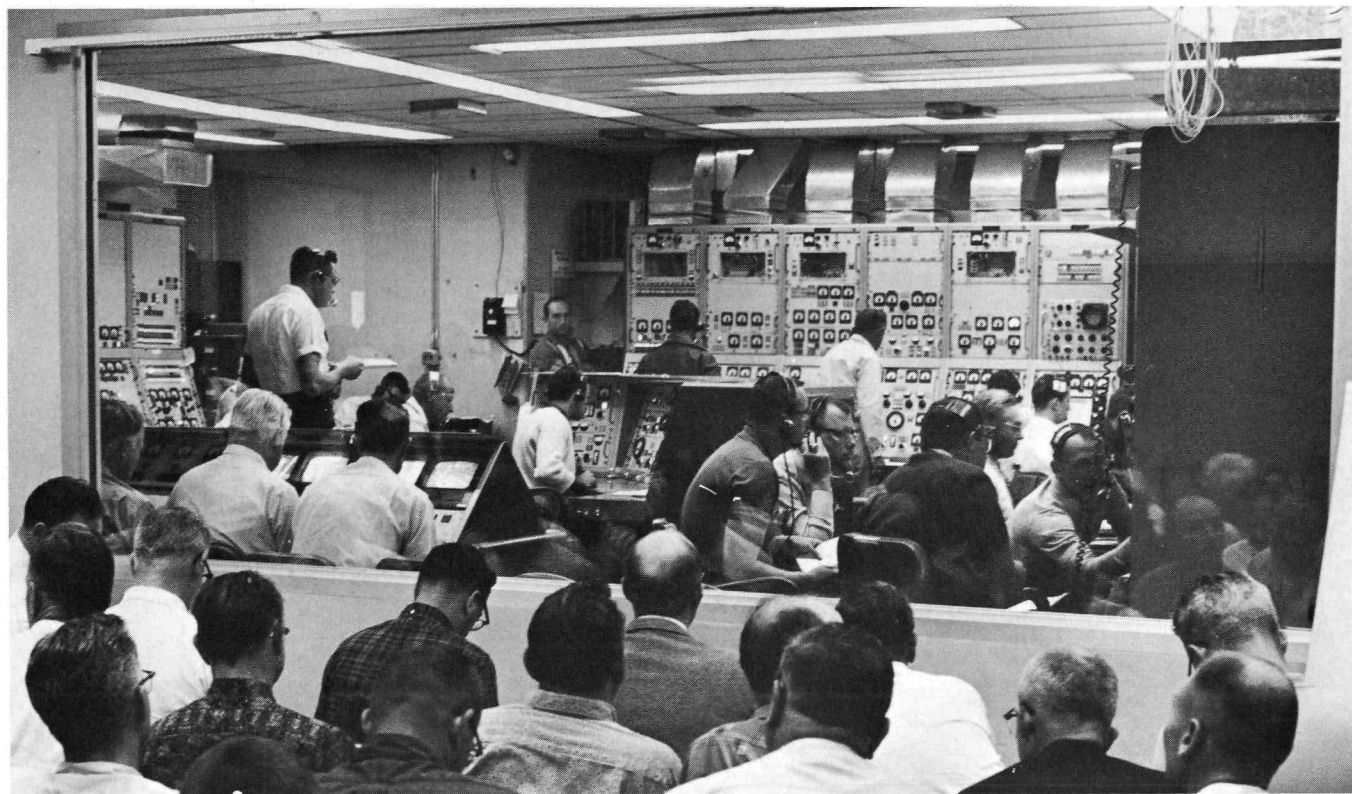
Interest mounts high as technicians and engineers monitor a space propulsion test in the Reactor Control building at the Nuclear Rocket Development Station, Nevada. Instruments record performance data.
