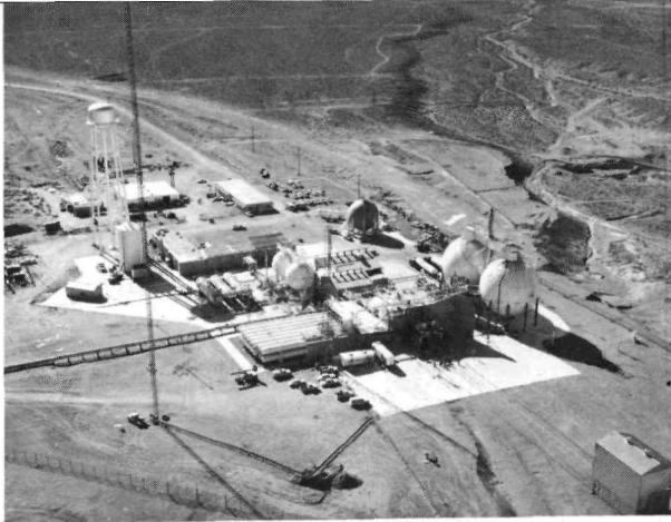
Test Cell C in 1967. Movable shields on test stand, right center, surround reactors during test. Building, lower right, can be moved on rails over reactors for weather protection.
