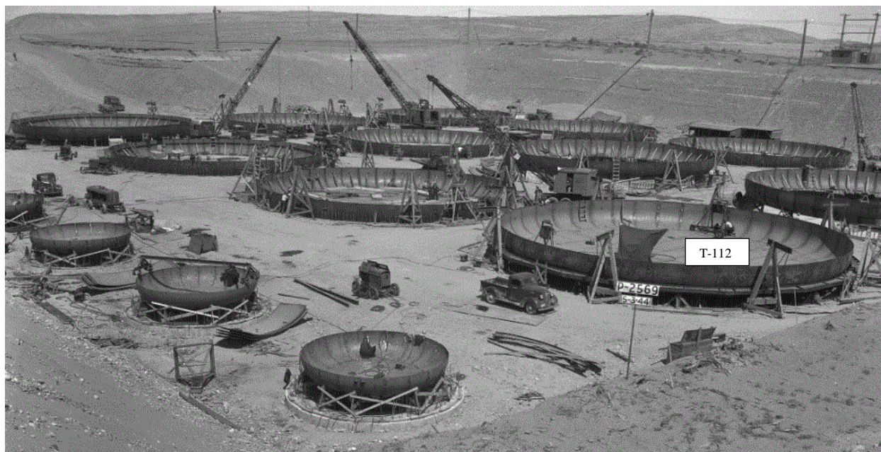
Figure B-5. Tank T-112 Bottom Liner and Knuckle Replaced Several Tanks Lowered with Bottom Liners Removed, Knuckles in Place May 3, 1944 (P-2569)
