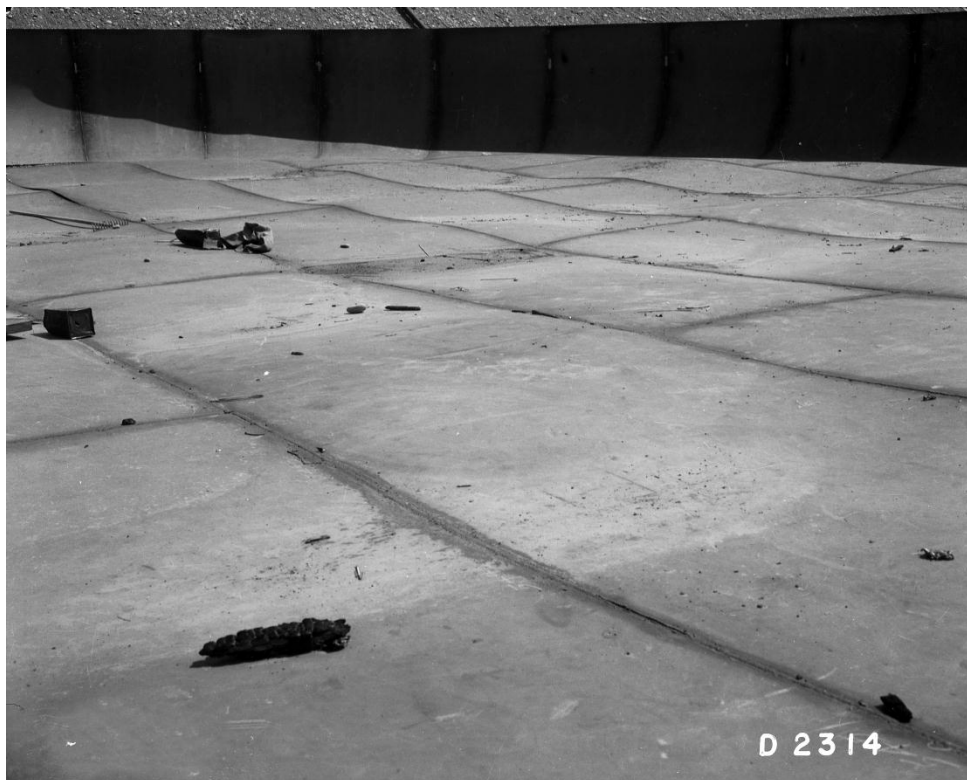
Figure 3-3. T Farm Tank Buckled Liner April 15, 1944 (Specific Tank Not Identified)
