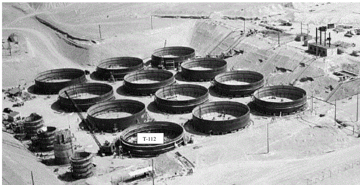
Tank T-112 identified for reference. Tank T-112 sidewalls being installed but tank was lowered before June 5, 1944, indicating bottom liner replacement was complete before that date. Other tanks appear to be lowered onto concrete pads indicating no further work on replacement bottom liners.
