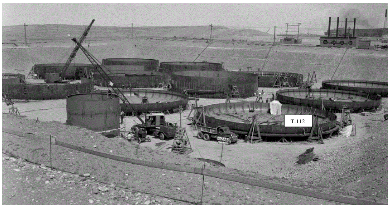
Figure B-6. T Farm Bottom Liner Repairs in Place Eight Tanks with at Least One Tier of Sidewalls in Place May 18, 1944 (P-2760)
