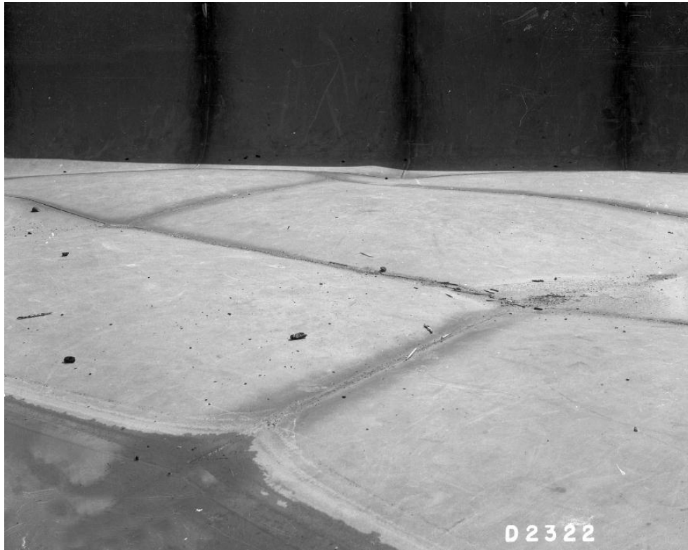
Figure 3-4. Tank T-111 Tank Buckled Liner April 15, 1944
