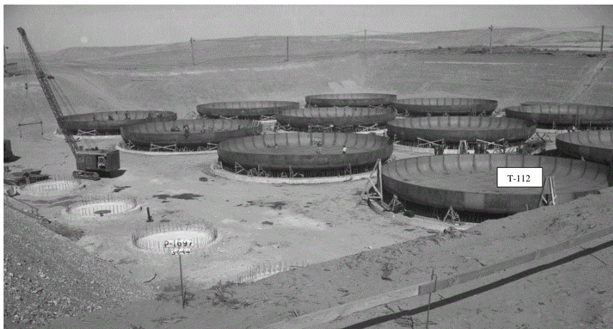
Figure B-2. All T Farm 100 Series Tank Bottom Liner and Knuckles Fabricated March 6, 1944 (P-1697)
