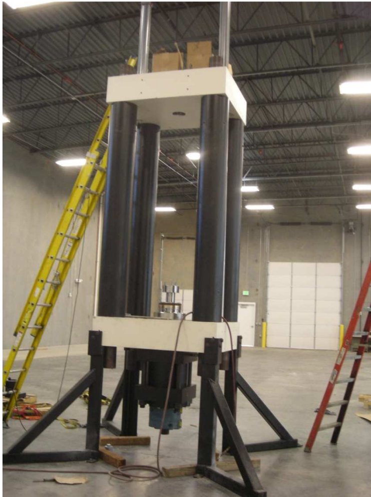
Figure 7 Picture Showing Construction of the UDS Load Frame
