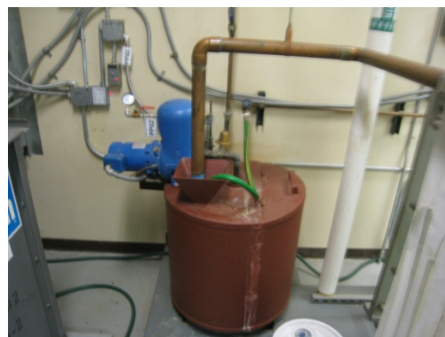
6 gallon Water heater installed in the Store.
