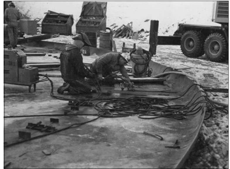
Welding Tank AY-102 Secondary Tank Bottom (8051-1-Photo)
