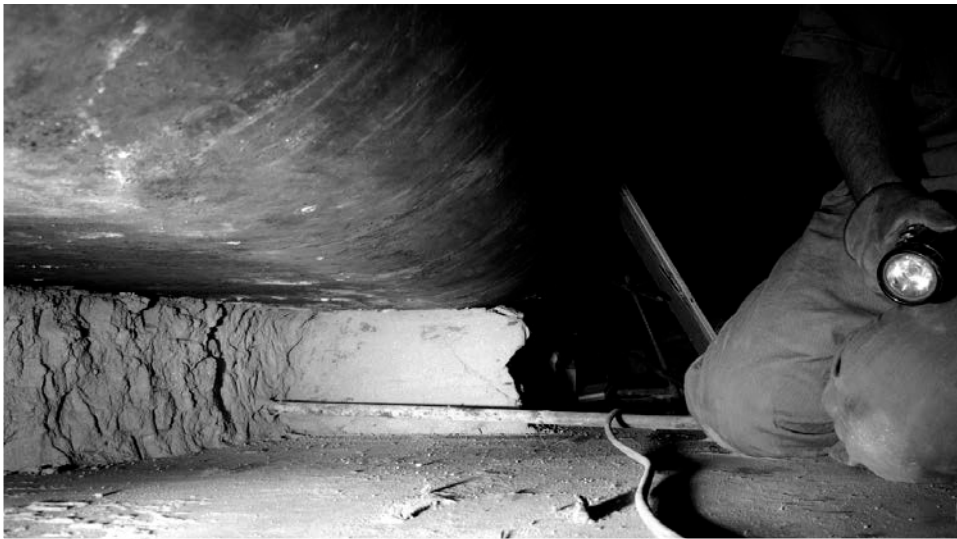
Preparing Insulating Refractory for modification with use of reinforced concrete
