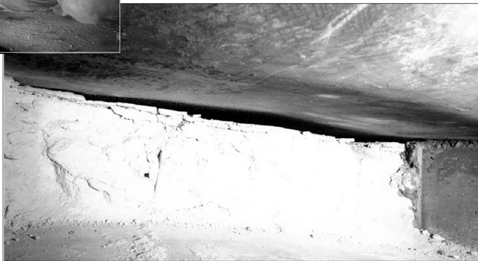
Tank AY-101 Primary Tank Gap over Insulating Refractory (52788-8-Photo). Gaps in Tank AY-102 were reported to be larger.
