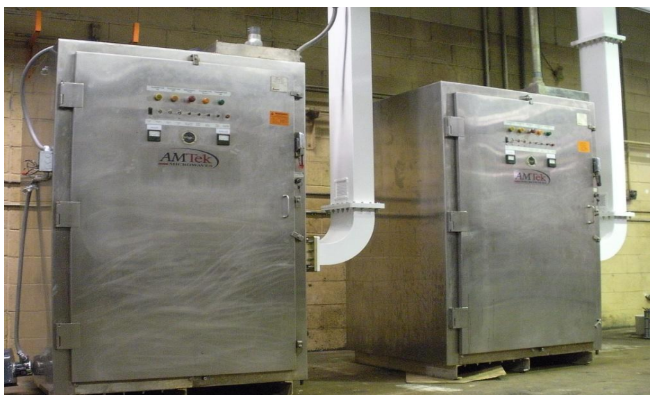
Figure 2: Two 75 kW Microwave Transmitters
