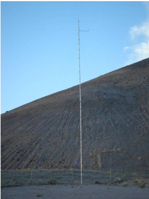
Figure 3. 20 meter NRG tower installed at the Barrick Mine site parking lot.
