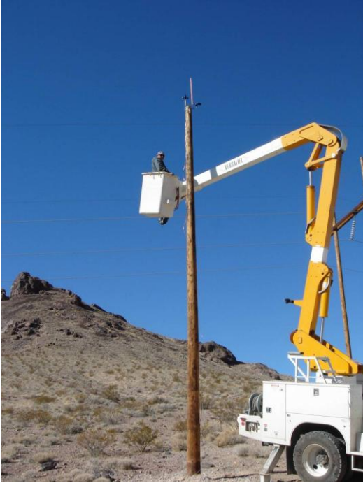
Figure 2. Danny Rogers, Lead Lineman at Valley Electric Association in Beatty, installing the station equipment atop a dedicated power pole at the Power Pole Site.
