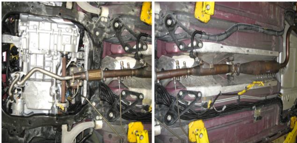
Figure 80: Initial Active Urea System Installed in the Development Vehicle
