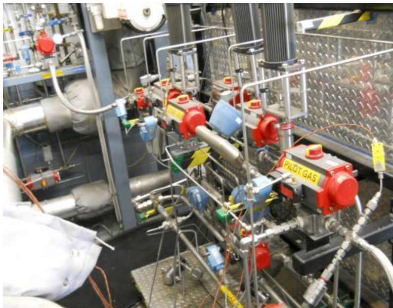
Figure 6(c). Solar Turbines, Incorporated Test Facility Showing the H 2 -N 2 -Pilot Fuel Skid with Filters and Emergency Stops
