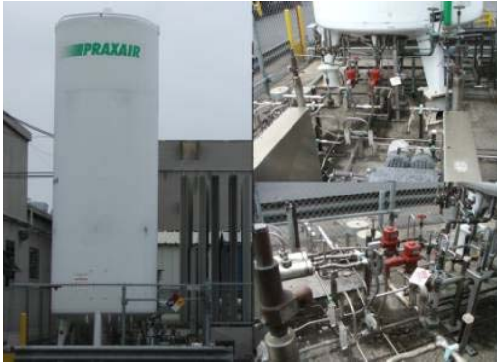
Figure 6(a). Solar Turbines, Incorporated Test Facility Setup Showing the N 2 Supply Tank and the Supply Lines
