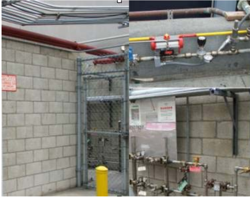
Figure 6 (b). Solar Turbines, Incorporated Test Facility Setup Showing the On-Off Valves for Start-Up and Shut Down for Safety
