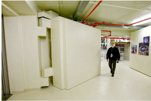
FIG. 2. One of 44 shield doors installed at the NIF.
