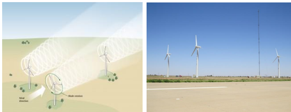
Figure 1: Scaled Wind Farm Technology Facility concept (left) and completed construction (right).
