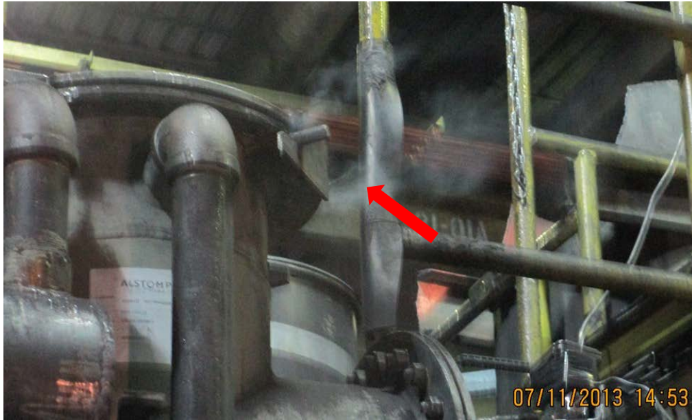
Fig 12. Smoke comes out of the cap of the tee section
