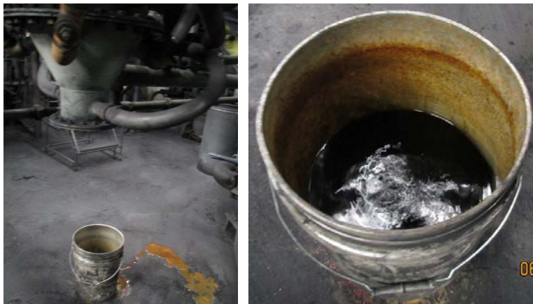
(a) Bottom cone of the afterburner collecting water
