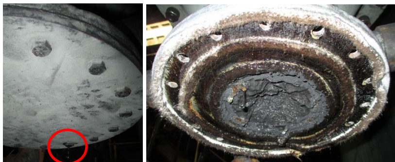
(b) Water dripping down and the mud like material in the cone section
