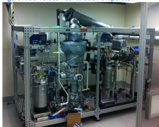
Figure A.11: Forced Recirculation Evaporator
