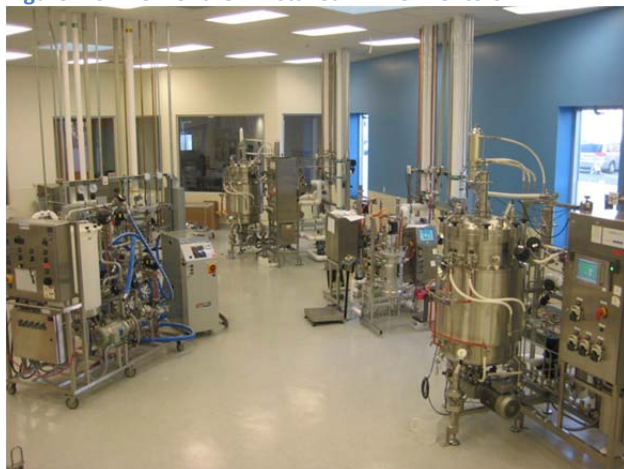
Figure A.9: View of the 2 Installed IBR Fermentors
