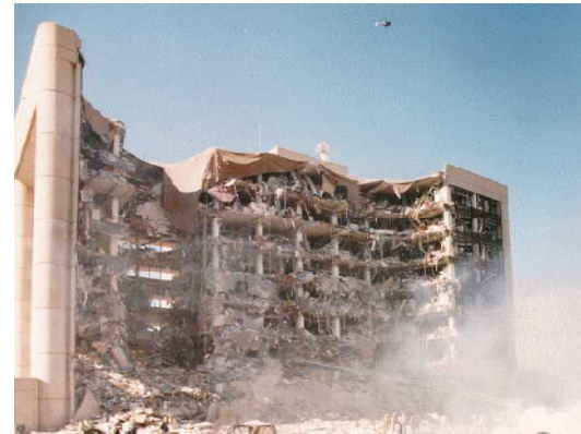
blast induced structural collapse
