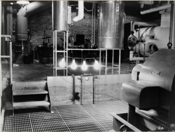
The first production of usable nuclear electricity occurred on 12/20/51, when four light bulbs were lit with electricity generated from the EBR-1 reactor.
