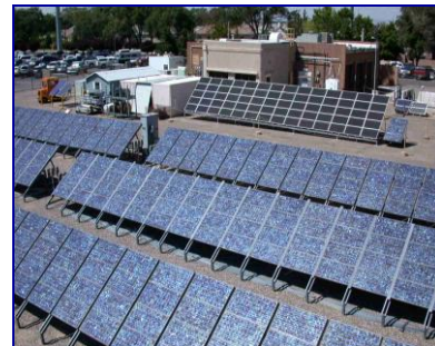
Figure 1 A portion of the PV arrays at DETL.
