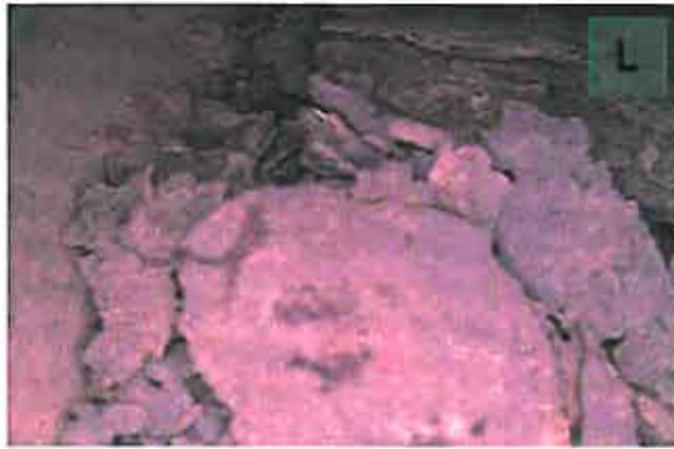
Figure 3-14. View of Debris on the Bottom of the Drain Line Just Prior to Entering Fourth Elbow (very dry)
