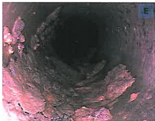
Figure 3-7. View of 6-in. Drain Line Part Way Between First and Second Elbow
