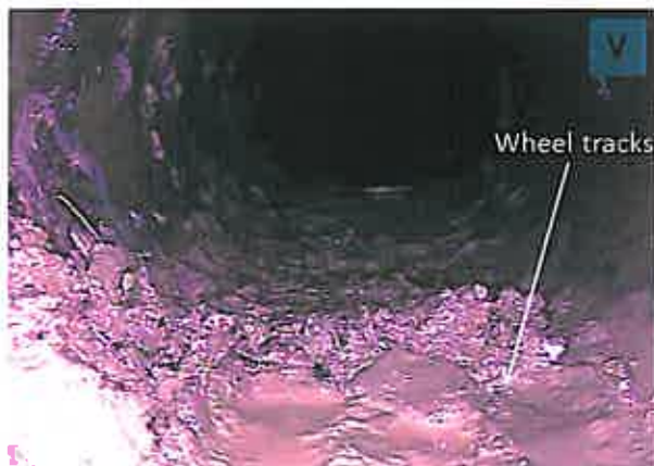
Figure 3-24. Partial View of the Saturated Debris on the Bottom of the Drain Line, Which Stopped Crawler Progress (approximately 7 ft from center of the tank)
