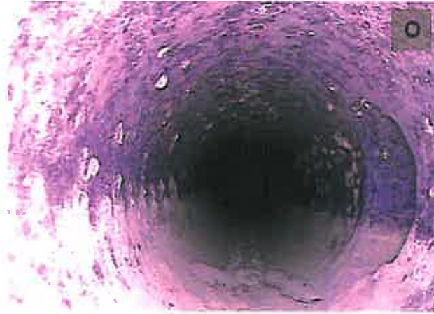
Figure 3-17. View of 4-in. Tee Entering the Side of the 6-in. Drain Line
