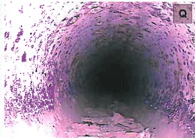
Figure 3-19. View of Debris on the Bottom of the Drain Line (about 2 ft from second tee)
