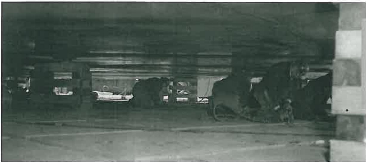
Figure 1-6. Workers Cleaning Debris from Foundation Drain Slots Prior to Lowering Secondary Tank Bottom (Photo 8096-1)
