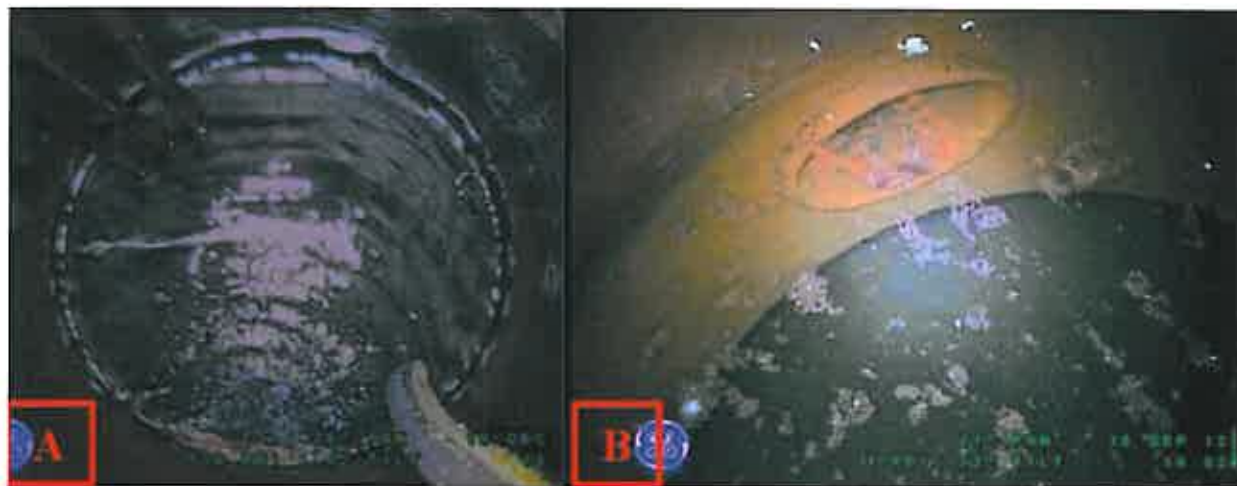
Figure 1-13. Photos from Video Showing Bubbling from Drain Line on 12/19/2012 (A), Photos from Video Showing Drain Line Just Underwater and No Bubbling on 9/18/2012 (B)
