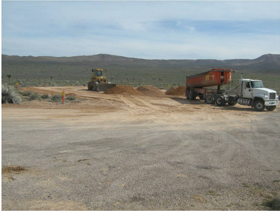
Photograph 5: Construction of the Cover at CAS 11-08-01, CWD #1, 03/28/2013
