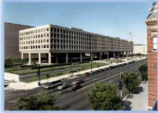
USG Initiates Project: January 2009
