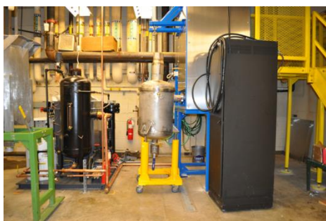
University of Washington High Pressure Steam Reactor and Dedicated Boiler
