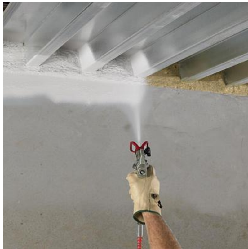
Protective spray insulation material for structural steel
