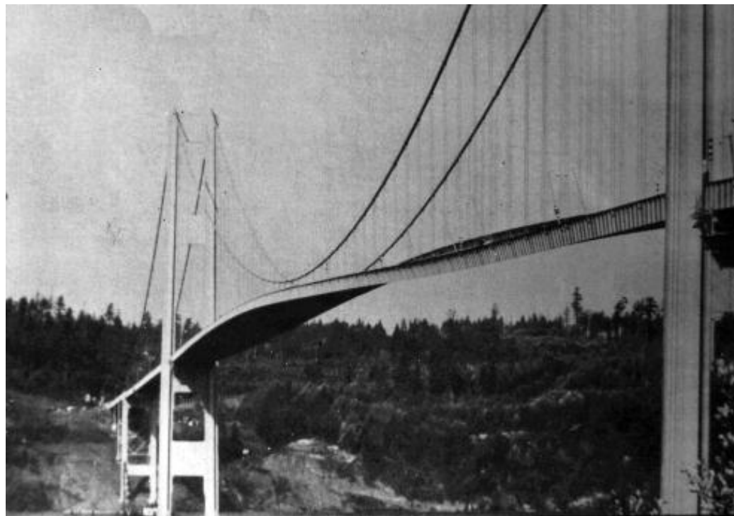
Tacoma Narrows Bridge Collapse:
