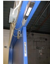
Flush Bolt, Magnetic Lock, and Balanced Magnetic Switch (door sensor)
