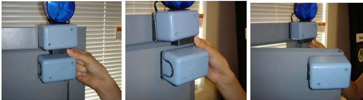
Figure 2: Reference Photos for Testing Balanced Magnetic Switch (BMS) Sensor with an External Magnet
