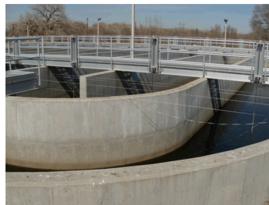
Chlorine contactor
