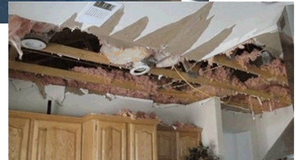
Water Damage Resulting from Burst Pipes
