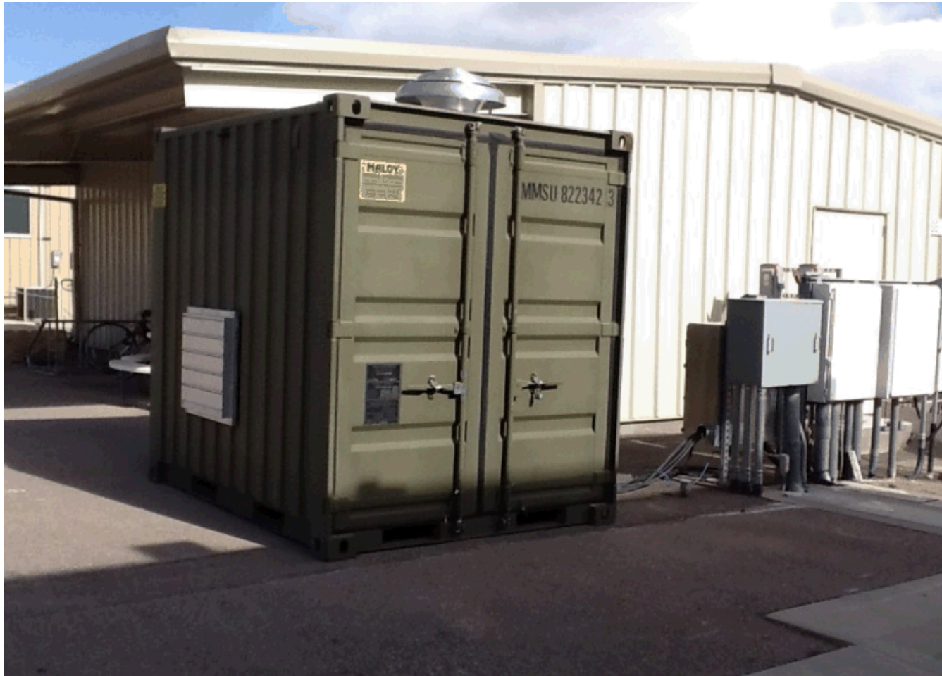
RK30 ESS: 30kW - 120kWh - Zinc Bromide Flow Batteries
