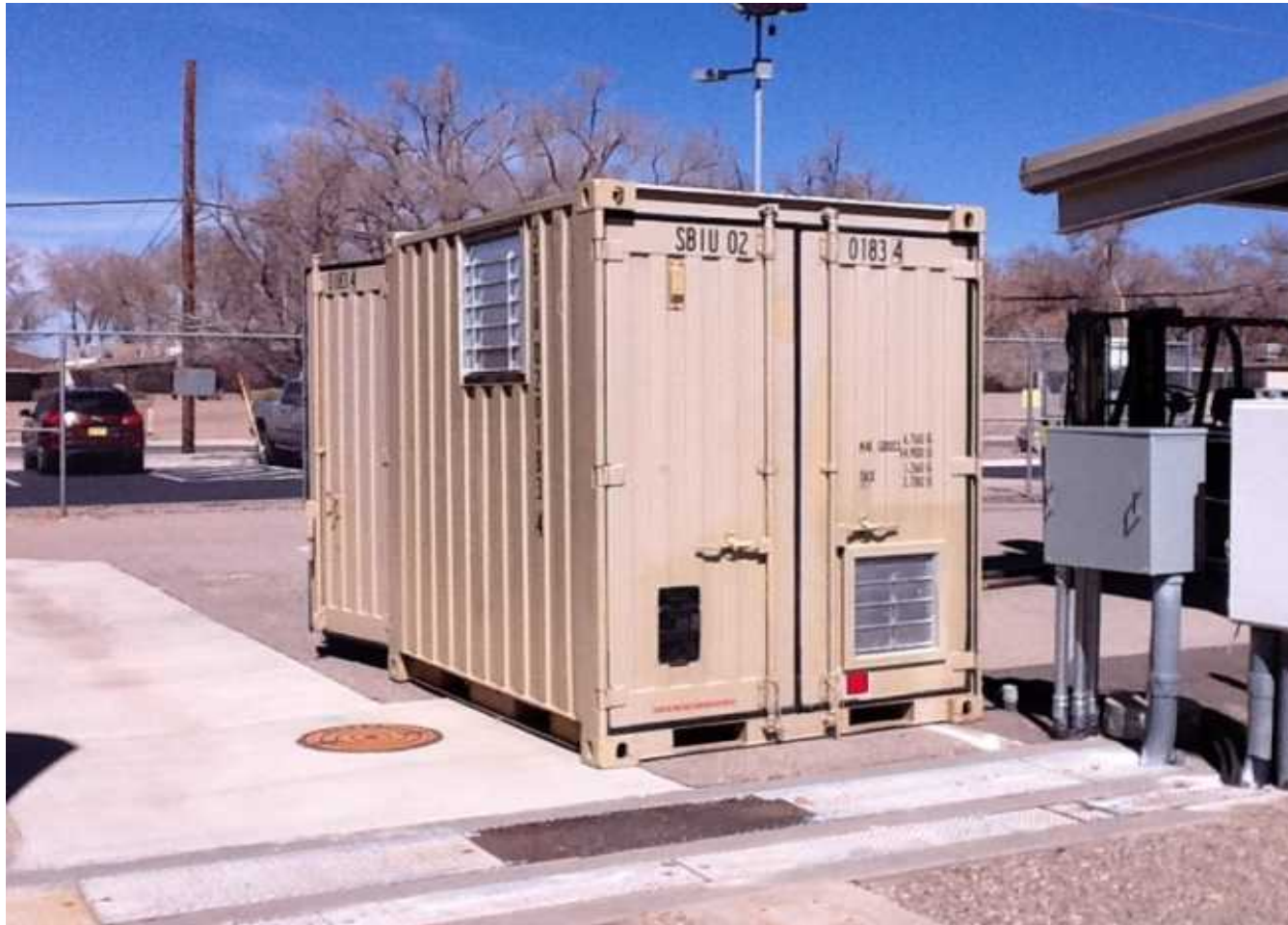
Prototype ESS: 100kW - 82kWh – Li-Ion Batteries
