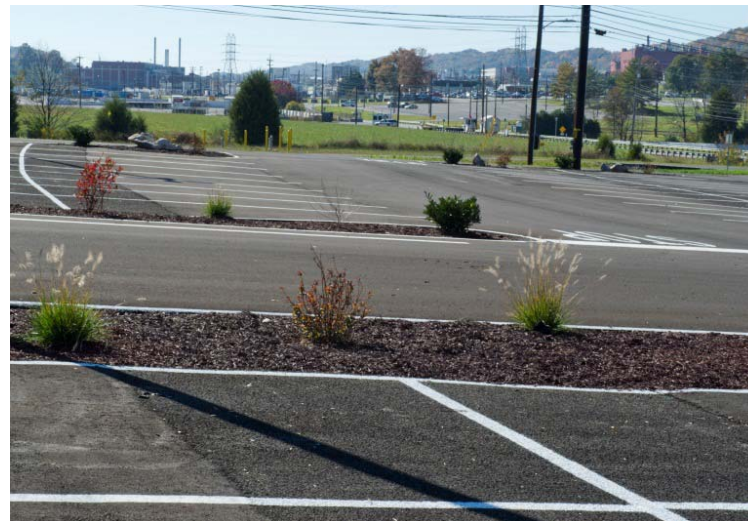
Fig. 4.2. (left) Faircloth Skimmer on UPF construction site. Fig. 4.3. (right) Pervious pavement and native planting contributes to EISA 438 requirements.
