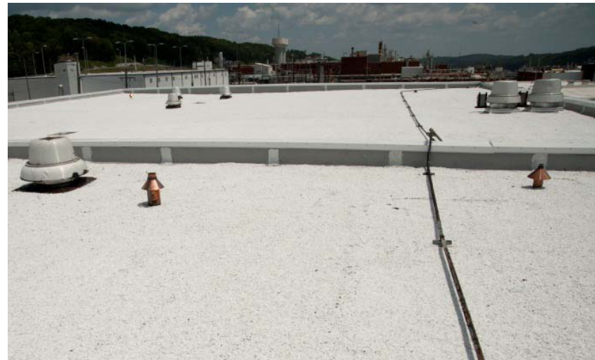
Fig. 2.5. 9103 cool roof installation.
