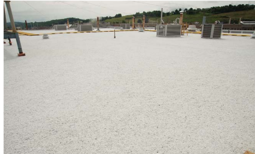
Fig. 2.4. 9204-02E cool roof installation.
