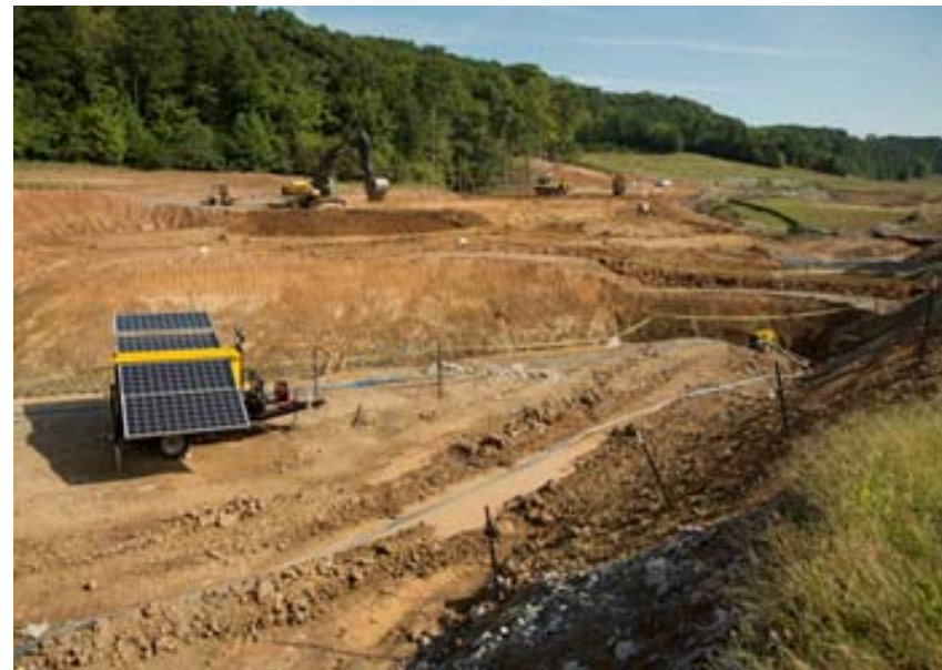
Fig. 8.1. Solar-powered generator on UPF construction site.
