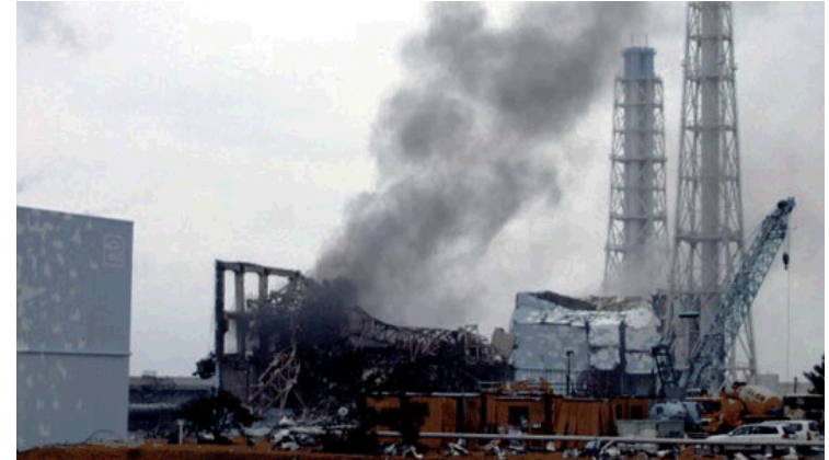
2011 Earthquake and Tsunami (Fukushima)
