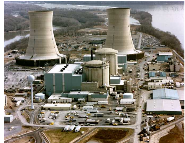
Nuclear Power Plant Cable Insulation
