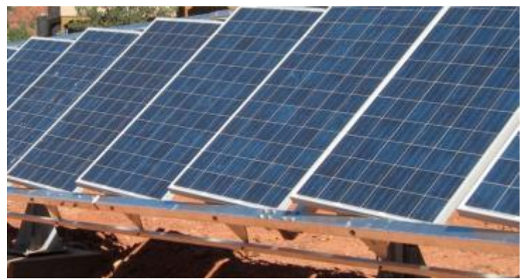
Low-cost, coarse 2-axis tracking with high acceptance angle and flat external surface
