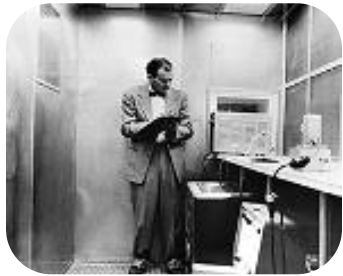
Laminar Flow Clean Room
