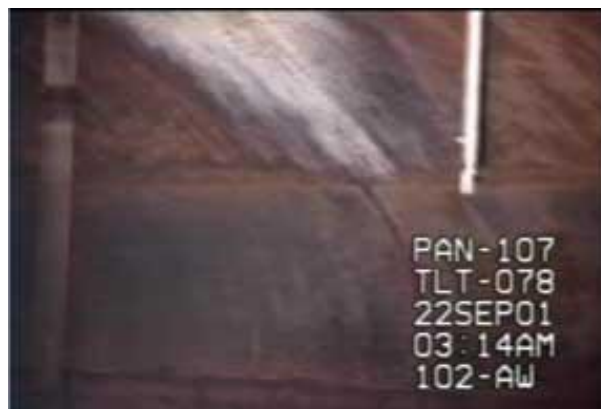
Figure 11. Tank AW-102 Dome White Deposit
