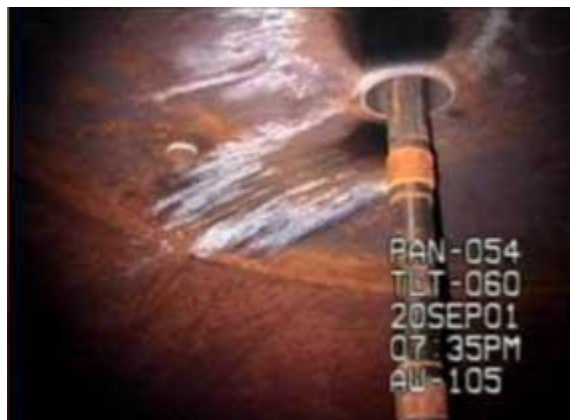
Figure 14. Tank AW-105 Dome White Deposits
