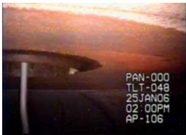
Figure 9. Tank AP-106 Dome Dollar Plate Corrosion
