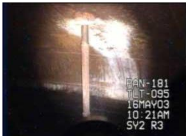
Figure 19. Tank SY-102 Dome White Deposits
