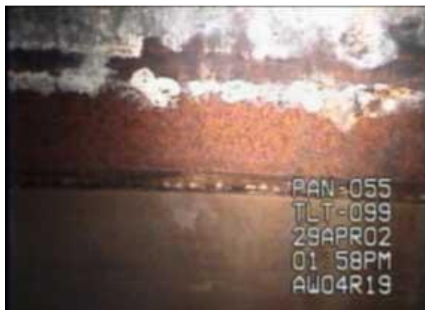
Figure 12. Tank AW-104 Dome Knuckle White Deposit
