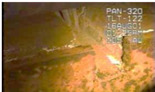
Figure 13. Tank AW-105 Refractory Degradation
