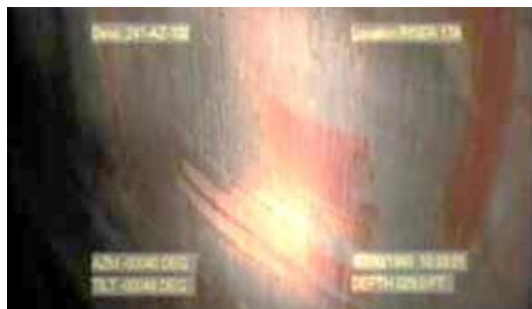
Figure 18. Tank AZ-102 Red Streaks on Wall of Primary Tank
