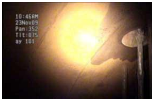
Figure 15. Tank AY-101 Dome Moisture
