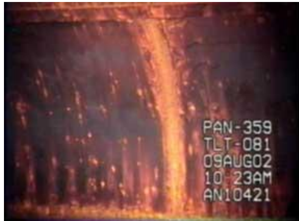
Figure 4. Tank AN-104 Dome Knuckle Bright Metal
