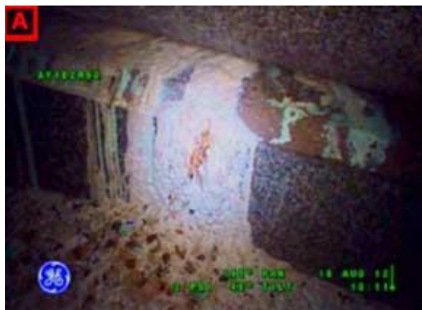
Figure 17. Tank AY-102 Tank Waste near Riser 90 in Annulus
