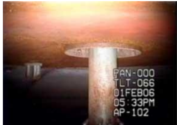
Figure 7. Tank AP-102 Dome Dollar Plate Corrosion
