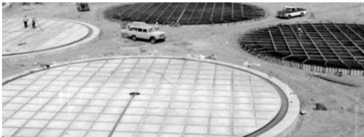
Figure 2. Tank Concrete Base Mat Construction
