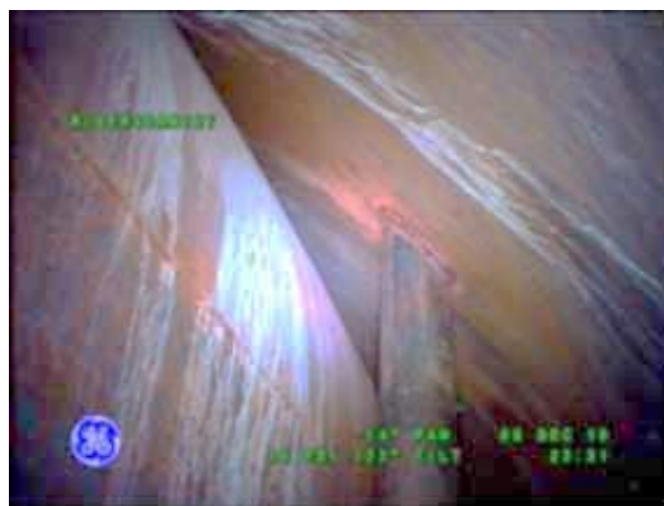
Figure 6. Tank AN-107 Top Knuckle Laitance Flow
