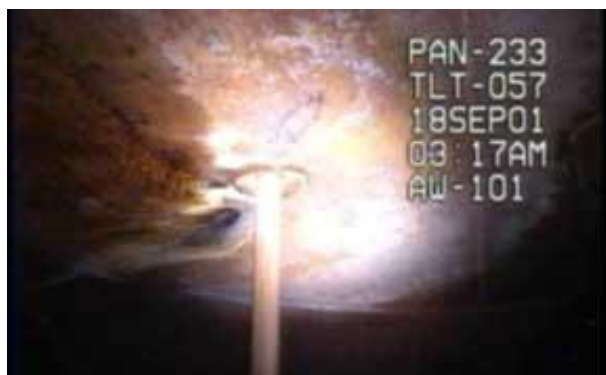
Figure 10. Tank AW-101 Dome Corrosion
