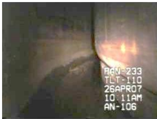
Figure 5. Tank AN-106 Annulus Floor Stain
