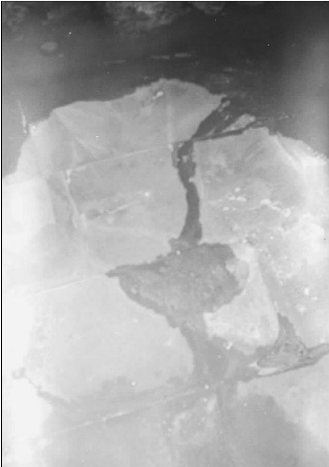
Figure 4-5. Tank U-104 Bulged Bottom Liner August 15, 1956 (Photograph 5BN1D0021185)
