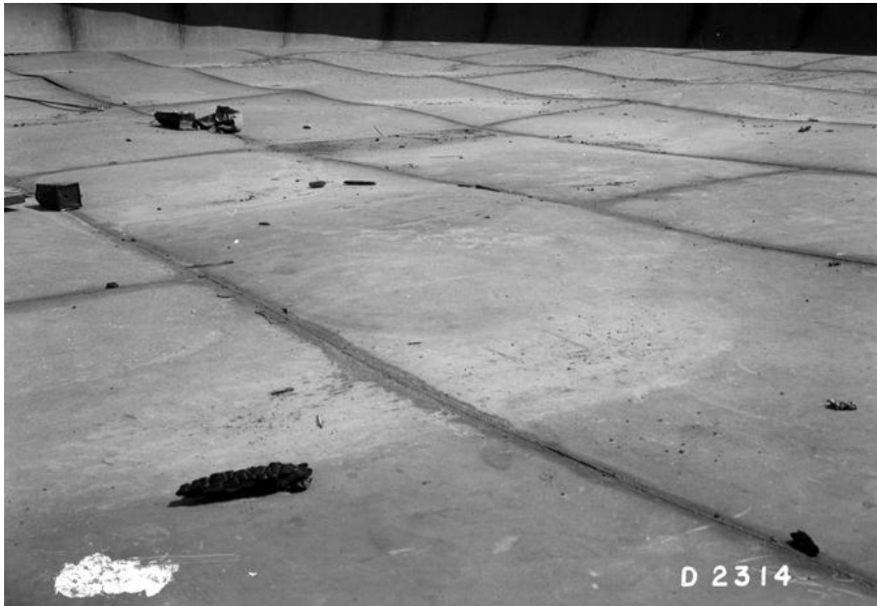
Figure 6-8. 241-T Farm Bottom Liner Deformation during Construction April 15, 1944 (D2314)
