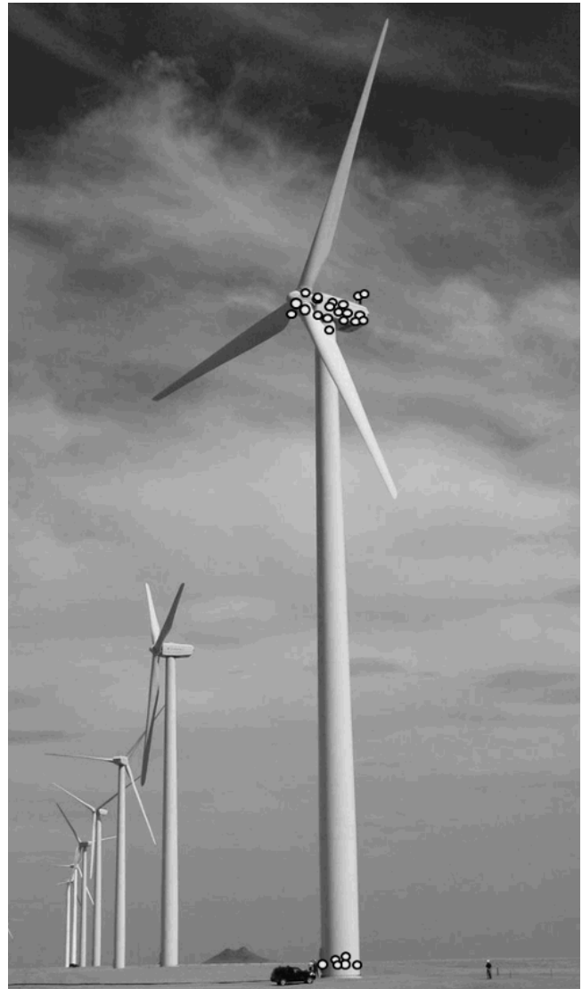
Figure 1: Annotated photo showing key sensor locations (hollow dots) in a typical utility-size wind turbine.
