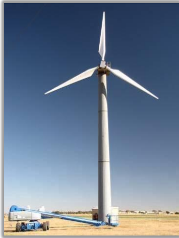
Micon turbine with 9m CX-100 blades
