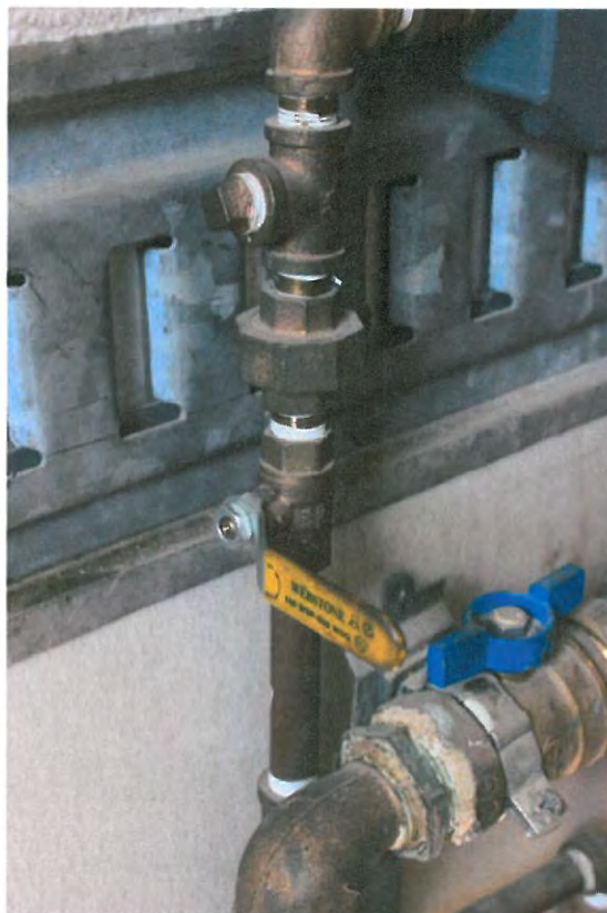
Figure B30: Nitrogen Pressure Control Valve
