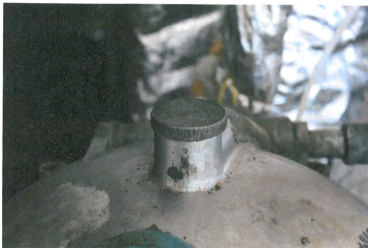
Figure B33: Top Threaded Plug in Prime Port
