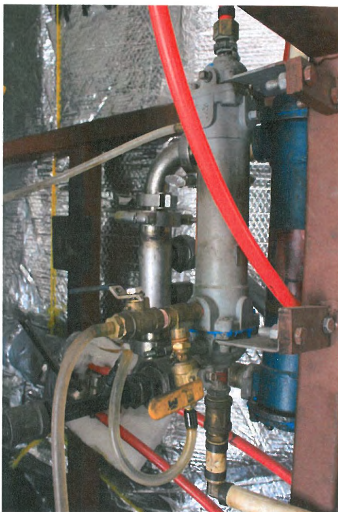
Figure B34: Water Line from Heat Exchanger
