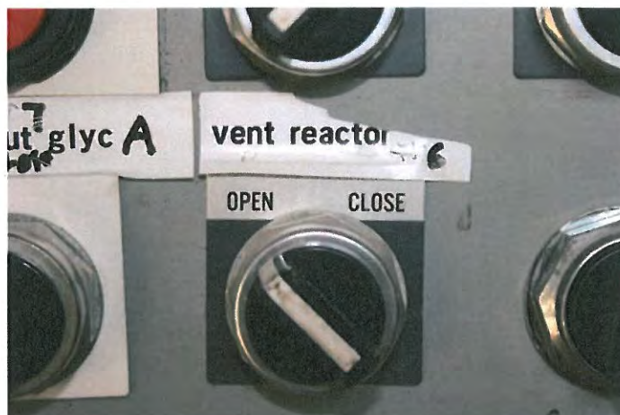
Figure B13: Reactor Vent Valve #6
