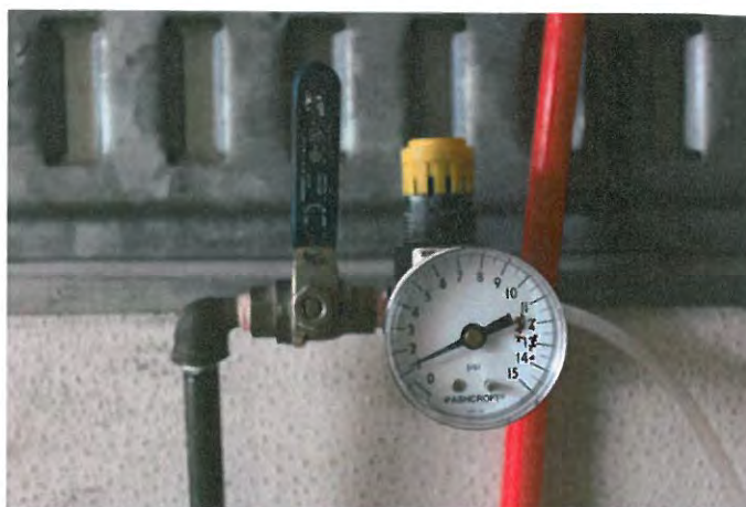
Figure B21: Nitrogen Pressure Regulator
