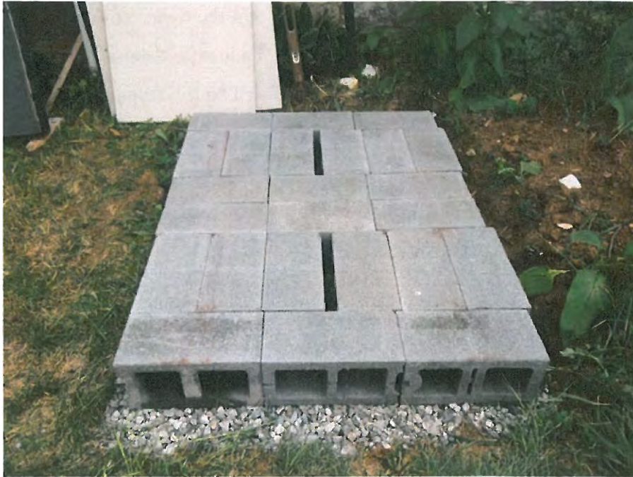
Figure 2: Foundation: involving 4-6 inch rectangular hole with leveled gravel and cinder blocks.
