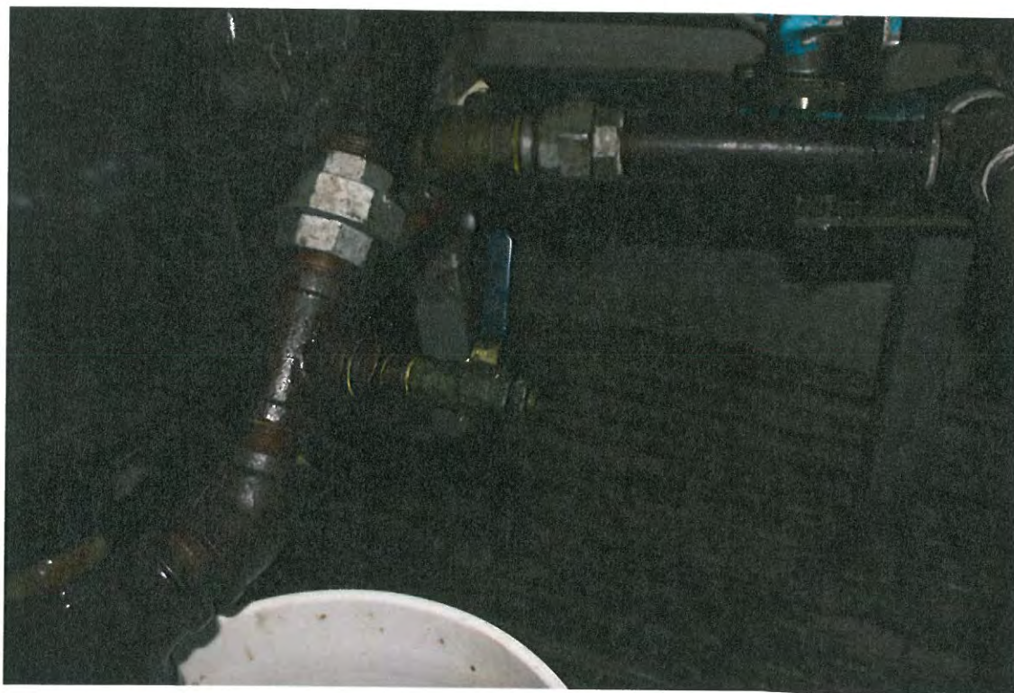
Figure B7: WVO Sample Valve in Trailer
