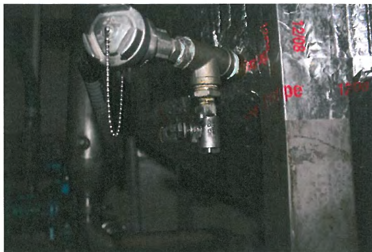
Figure B24: Reactor Sample Valve
