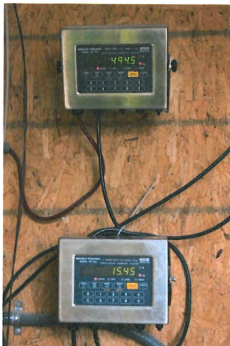
Figure B15: Mass Indicators for Reactor (top) and Potassium Methylate Vessel (bottom)
