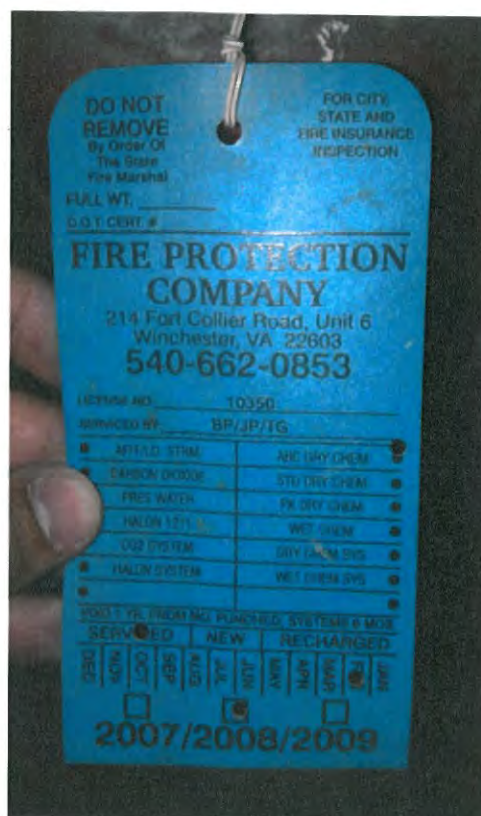
Figure A27: Expired Fire Extinguisher Tag
