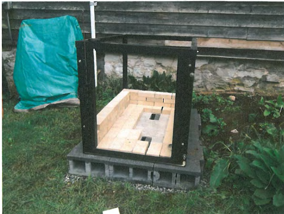
Figure 3: Steel frame and beginning of floor and brick wall
