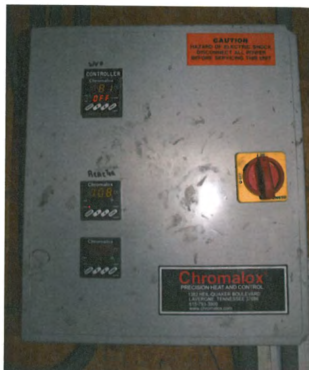
Figure B2: Tank Temperature Readouts
