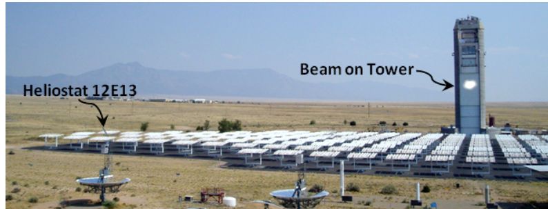
Fig. 2. Photograph of heliostat 12E13 at the NSTTF in Albuquerque, NM, focusing the sun onto the tower’s North face.
