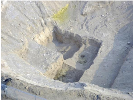
Maximum Excavation 30 ft bgs in one area
