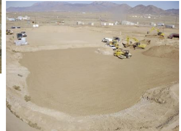
Backfill at ~8 ft bgs
