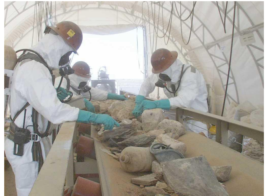
Conveyor System for Debris & Rock Segregation
