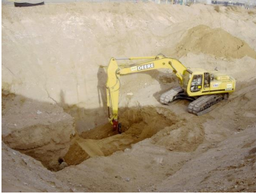
Excavation to 30 ft bgs for PCB-contaminated soil
