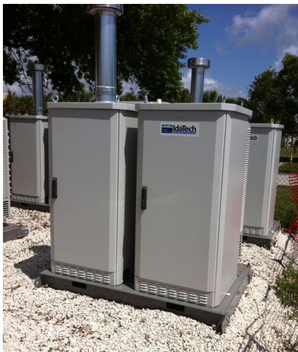
Figure 5.9 Close-up of an EVCS IdaTech FCS
