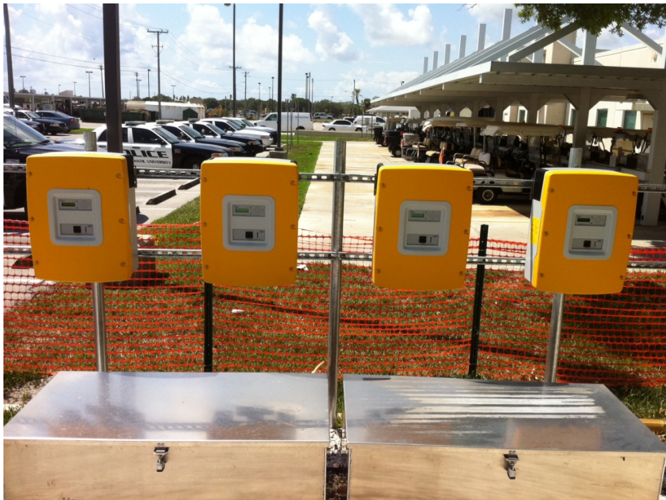
Figure 5.8 EVCS inverters and battery boxes with FAU EV charging complex in background
