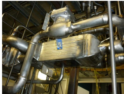
HEX320 Recycle Heat Exchanger
